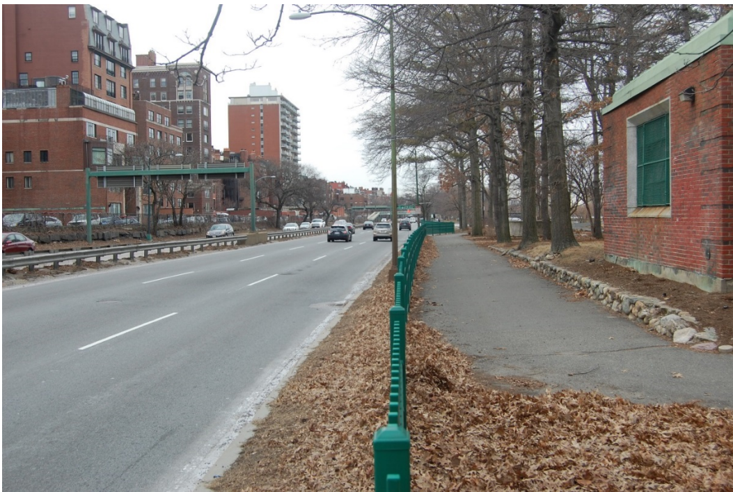
Existing Lights Photos – 2
