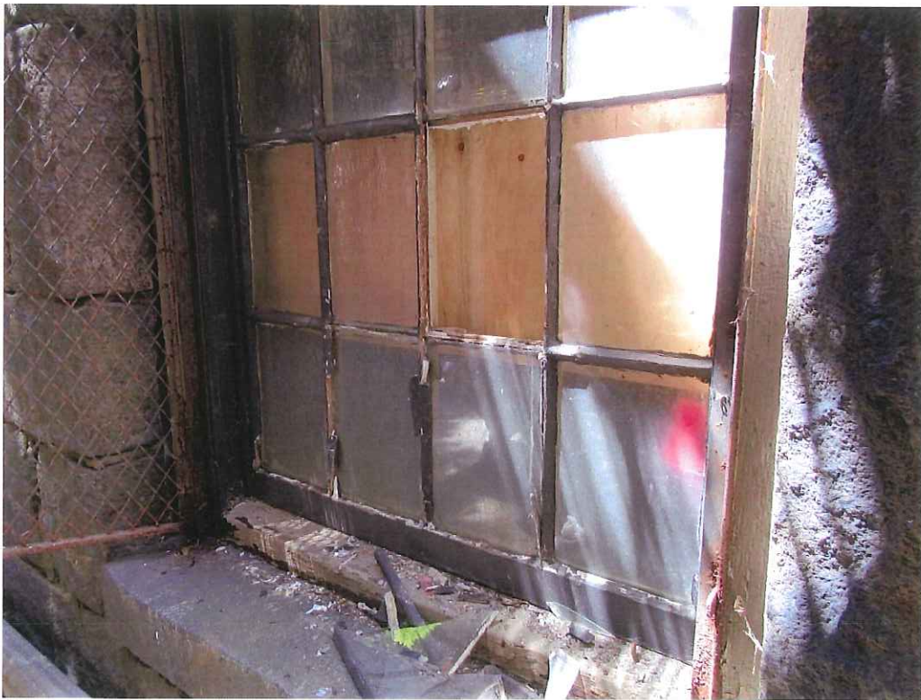
6. South elevation window, typical condition
