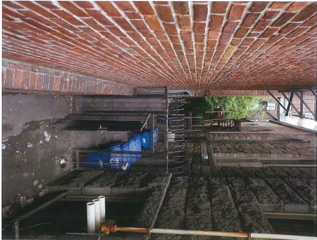
4. South elevation, view west with location of new gas meters and enclosure at far right
