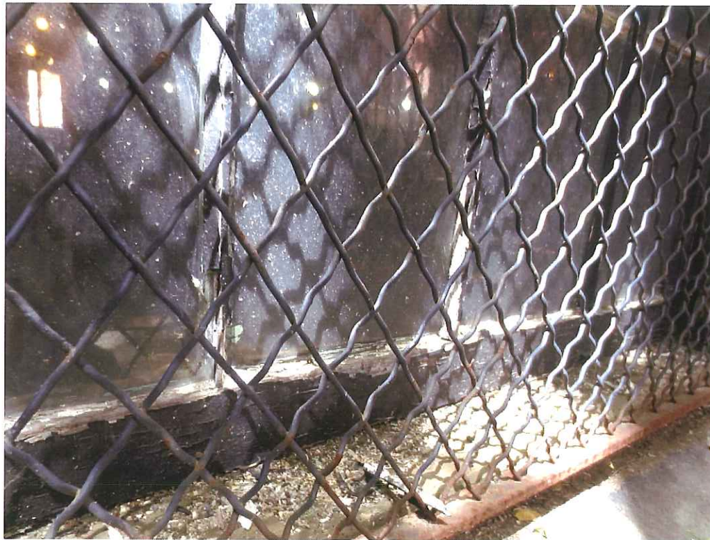
12. South elevation window, typical condition
