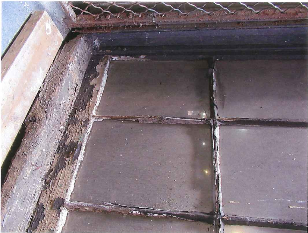
14. South elevation window, typical condition
