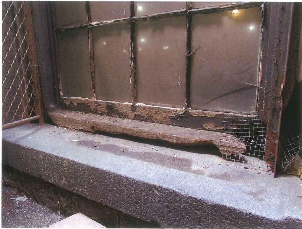
5. South elevation window, typical condition
