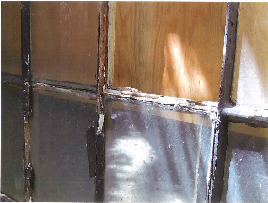
10. South elevation window, typical condition
