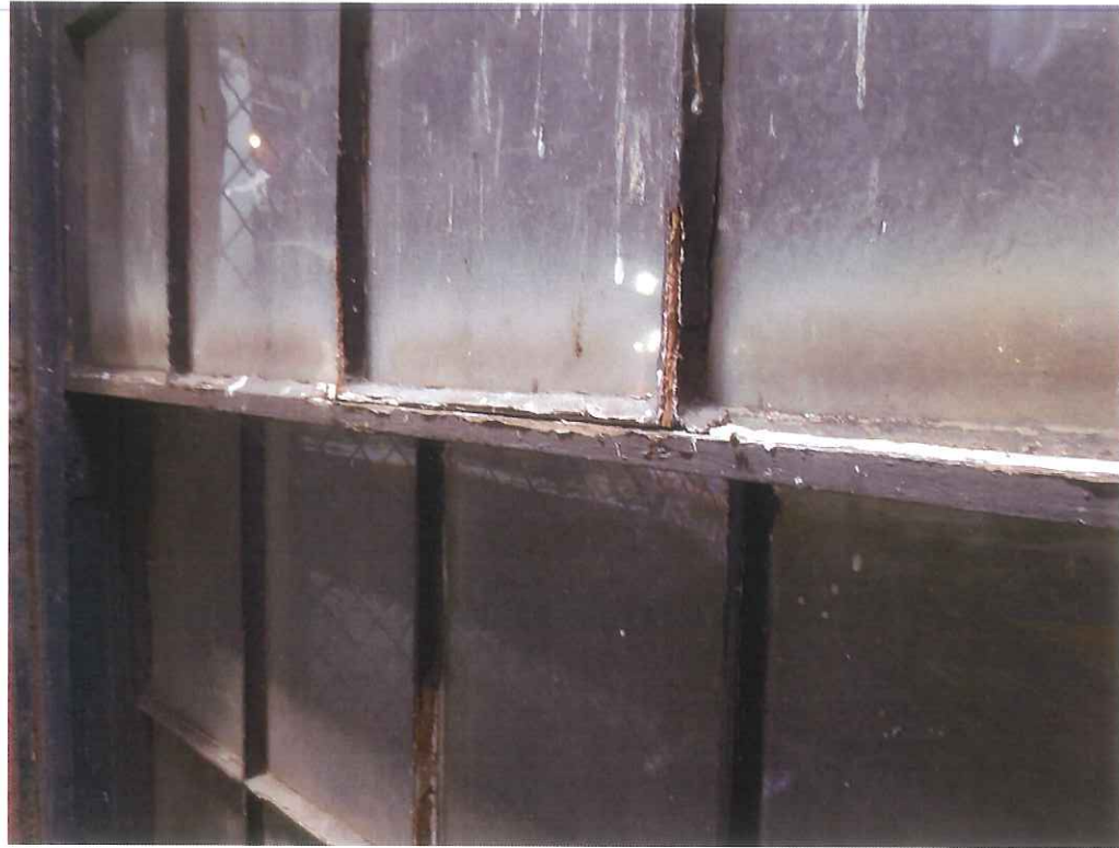
7. South elevation window, typical condition
