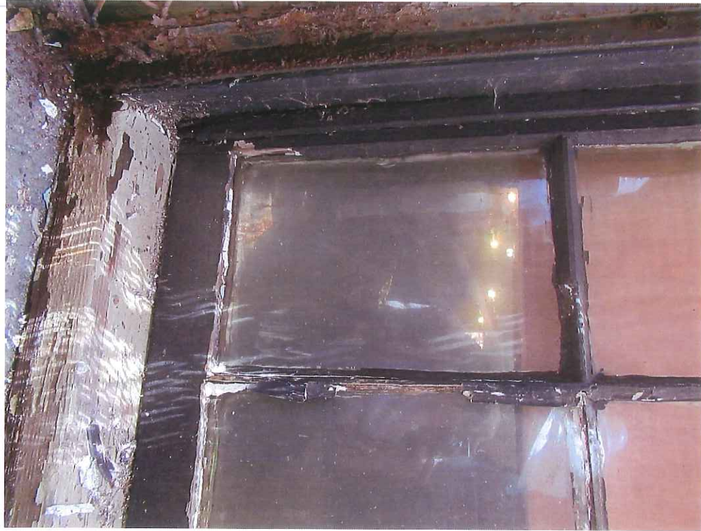
13. South elevation window, typical condition
