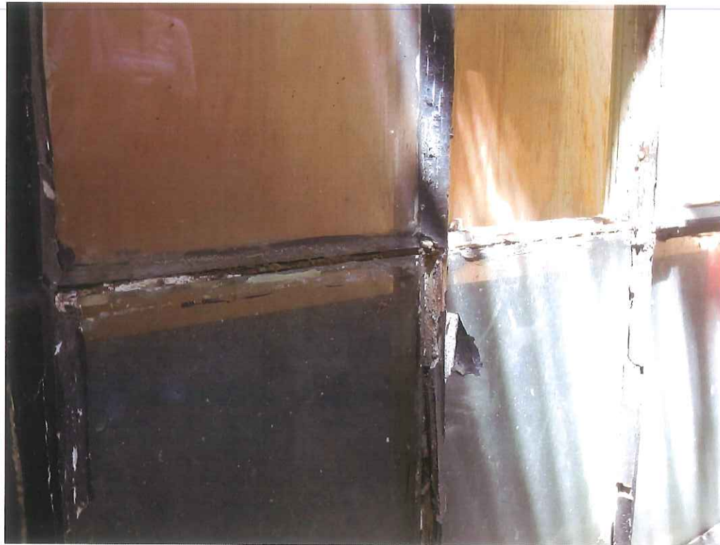
11. South elevation window, typical condition
