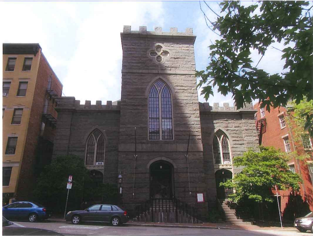
1. East elevation, view west from Bowdoin Street
