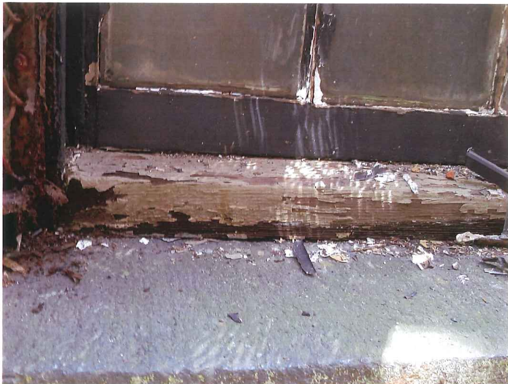
8. South elevation window, typical condition
