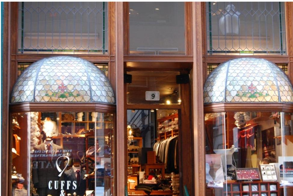
**Figure #15.** View of the stained glass elements and wood storefront at the Water Street elevation (looking south), October 2015.
