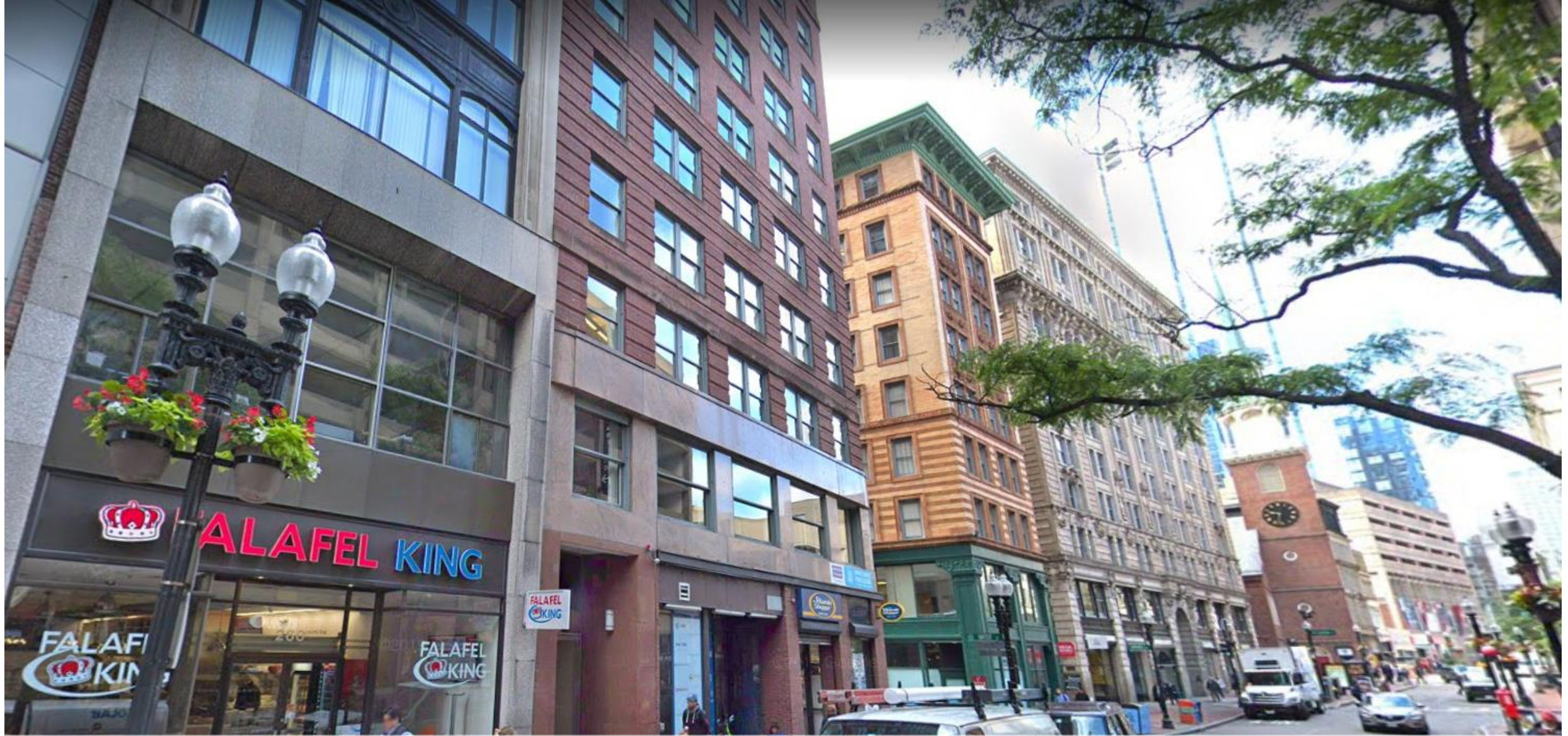
View from North from Washington Street
