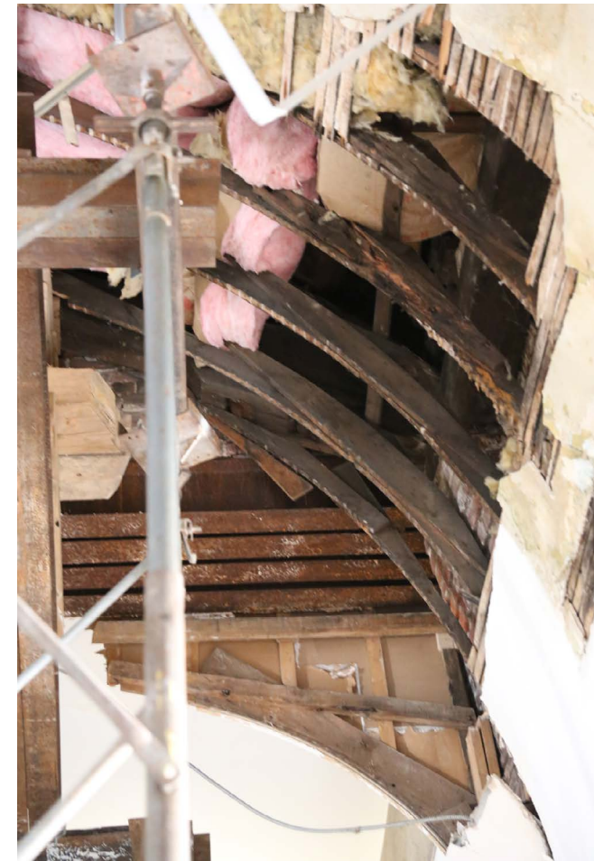
Probes and Shoring at roof framing (Spring 2019)
