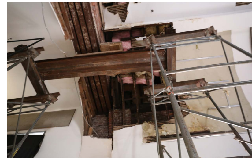
Tower and roof support shoring from below (Spring 2019)
