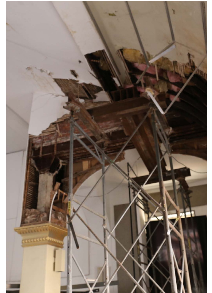
Interior tower shoring & reinforcement (Spring 2019)
