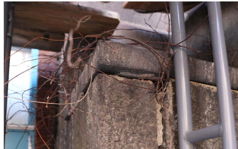
Stone displacement in granite base (Spring 2019)
