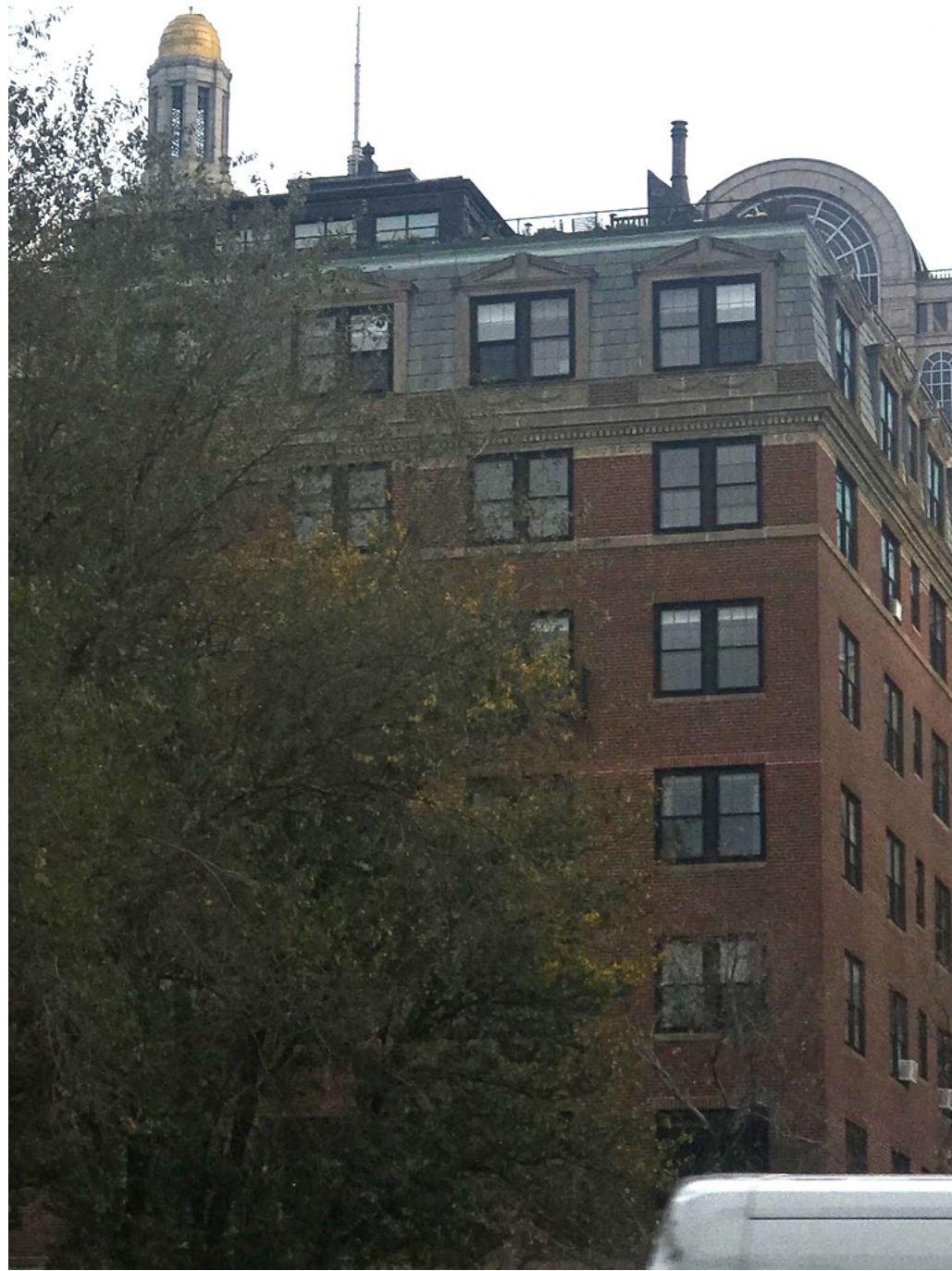
Clarendon Street Playground View 90 Commonwealth Avenue
