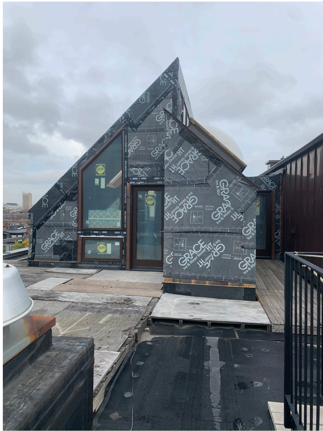
South View 90 Commonwealth Avenue, Unit 24 Penthouse & Deck
