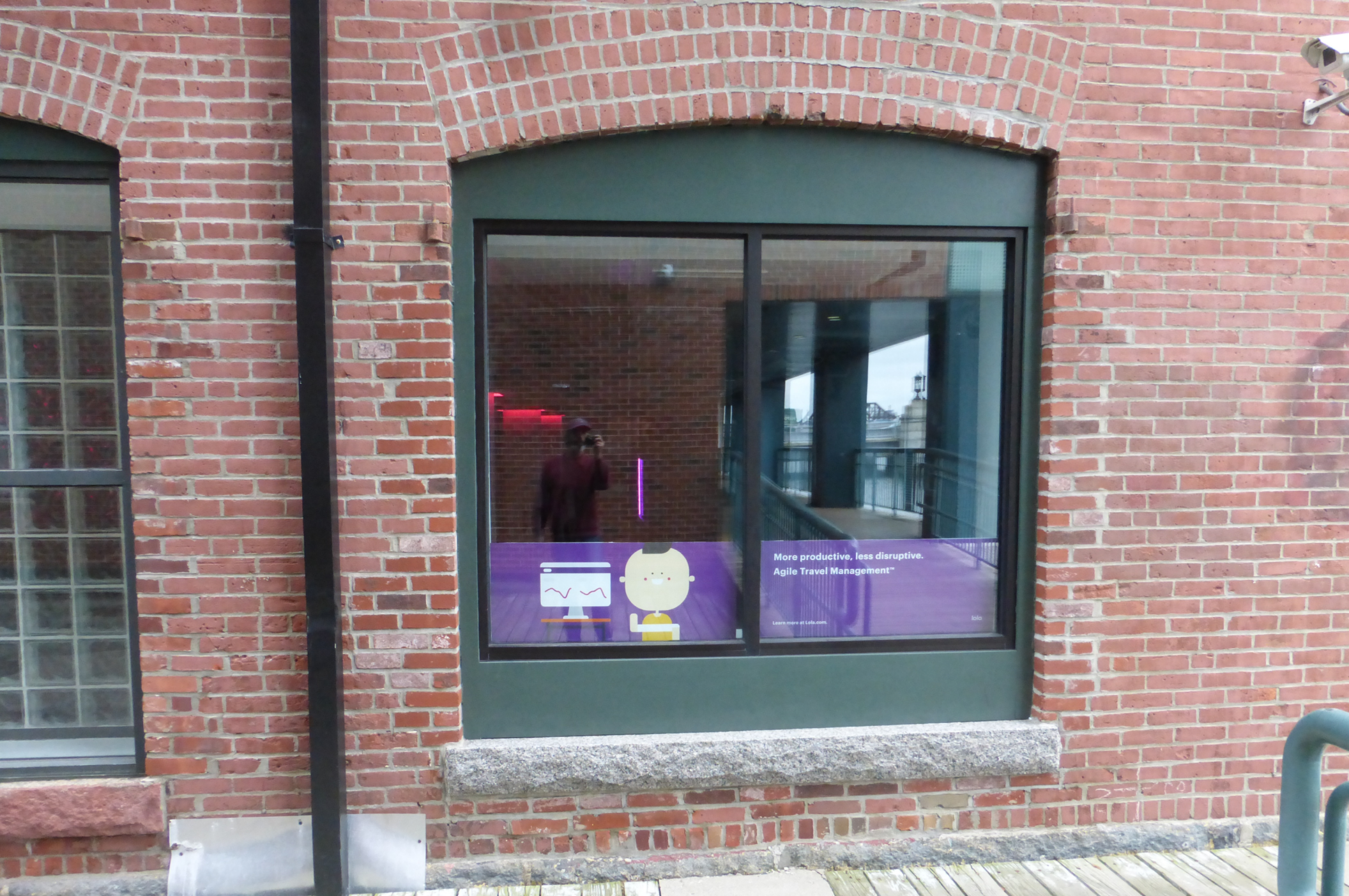
4. VIEW AT WINDOW AT GRADE - REAR OF BUILDING
