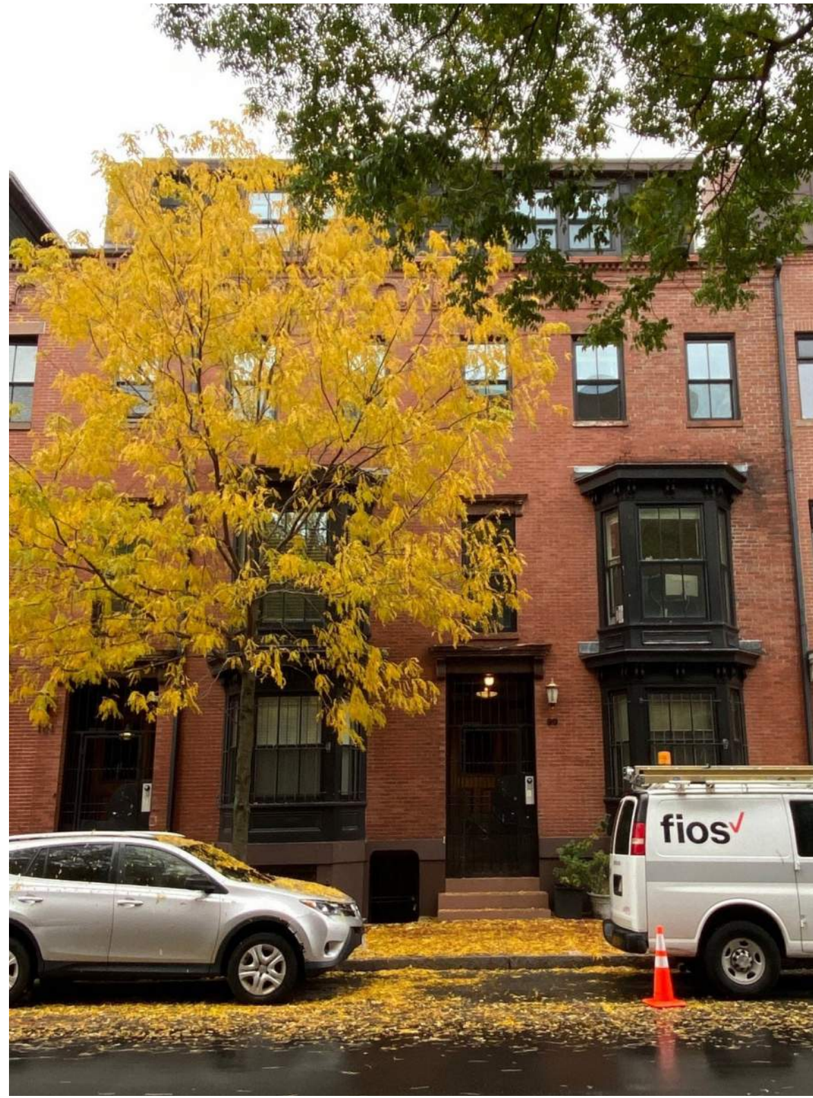
99 & 101 W. Springfield St. - In April 2012 replaced original windows and storms with new Jeld-Wen insulated glass windows with city approval
