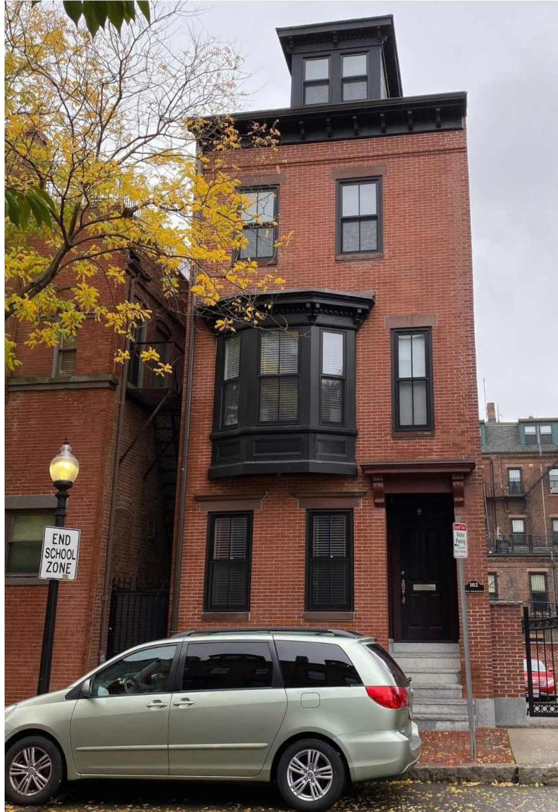
102 W. Springfield St. - In 2012 replaced original Chain and Pulley windows with new aluminum clad insulated glass windows with city approval
