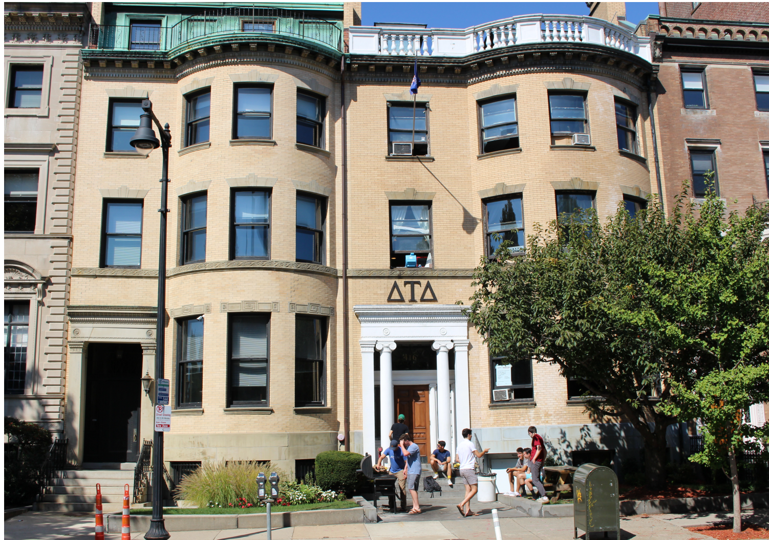
EXISTING FRONT FACADE
