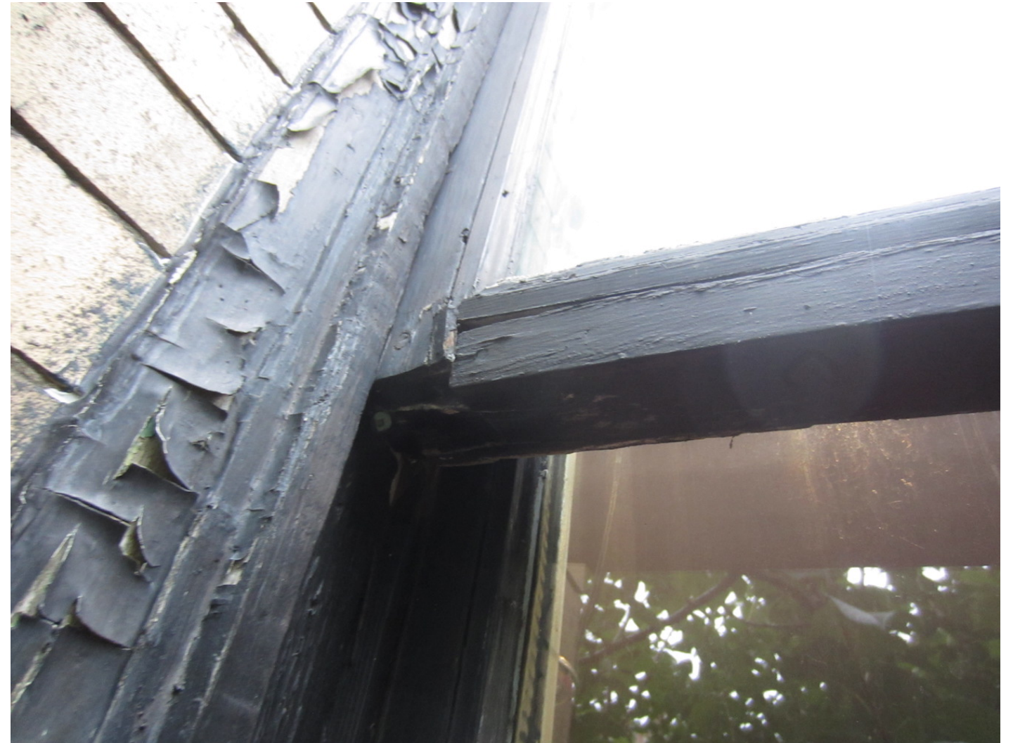
EXISTING WINDOW CONDITION (EXTERIOR FIRST FLOOR FRONT)
