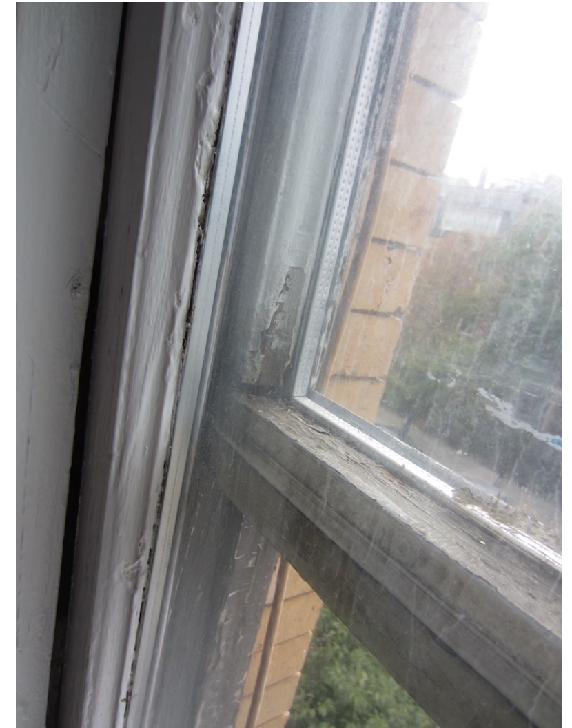
EXISTING WINDOW CONDITION (THIRD FLOOR FRONT RIGHT)
