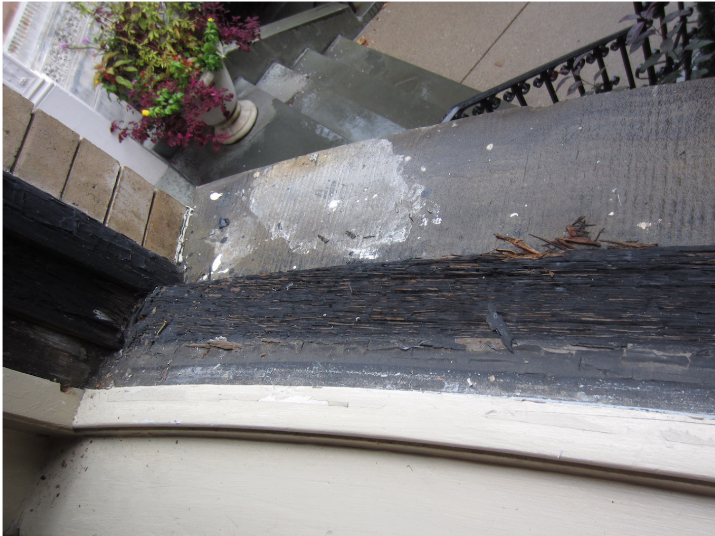
EXISTING WINDOW CONDITION (SILL FIRST FLOOR FRONT)
