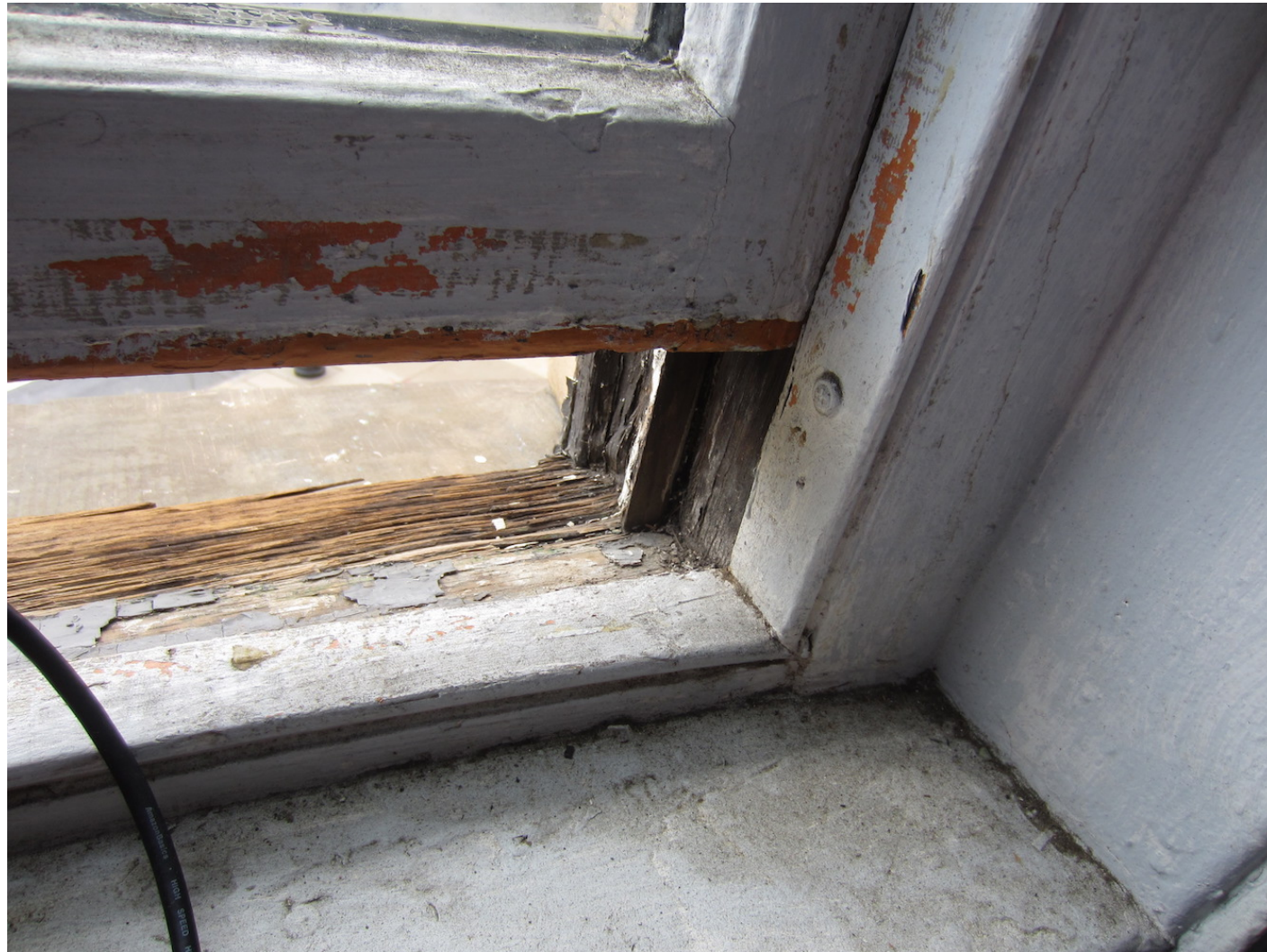
EXISTING WINDOW CONDITION (SILL SECOND FLOOR FRONT)
