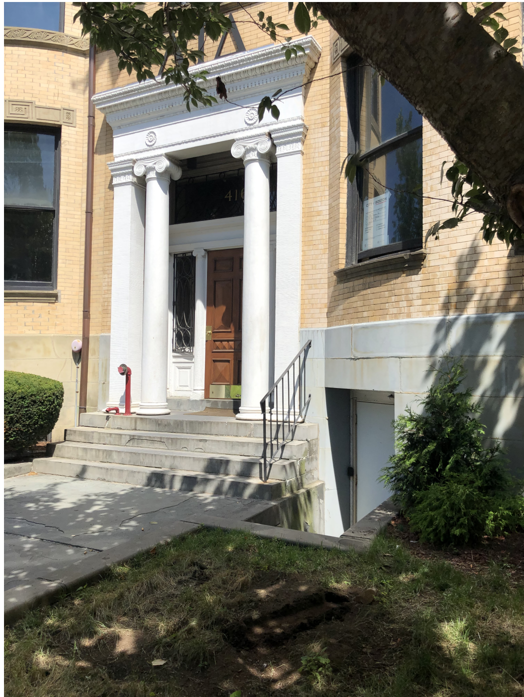
EXISTING FRONT ENTRANCE
