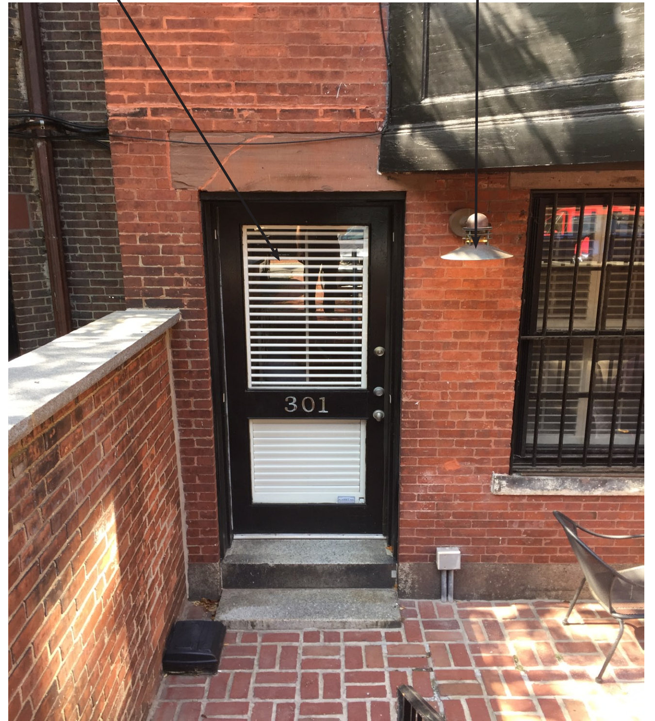
Removal of non-historic lighting fixture
