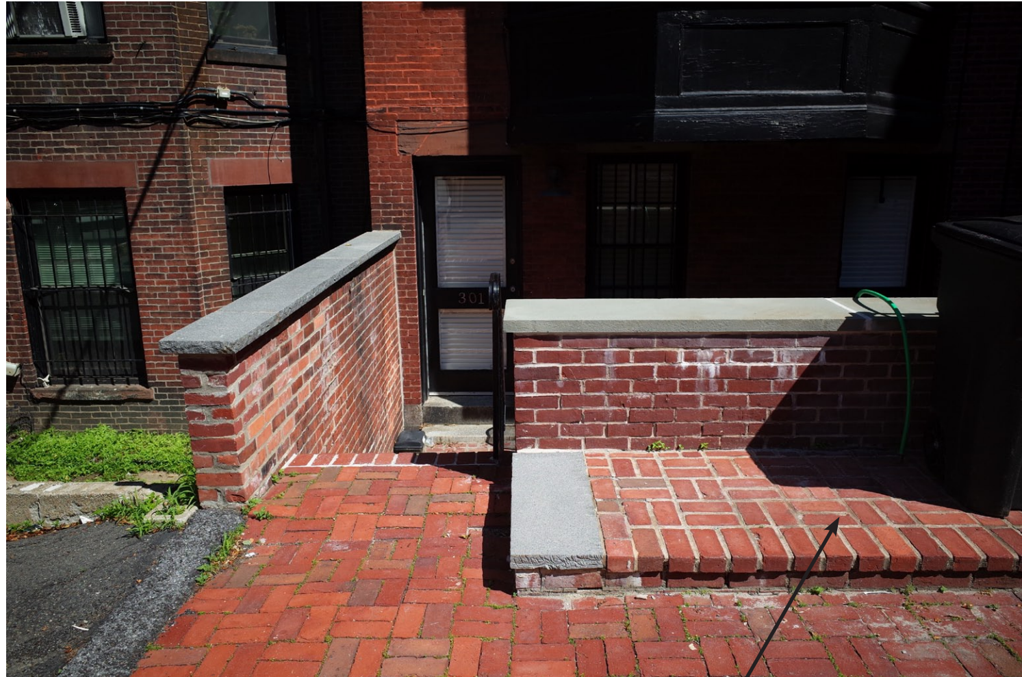
Removal of brick plinth
