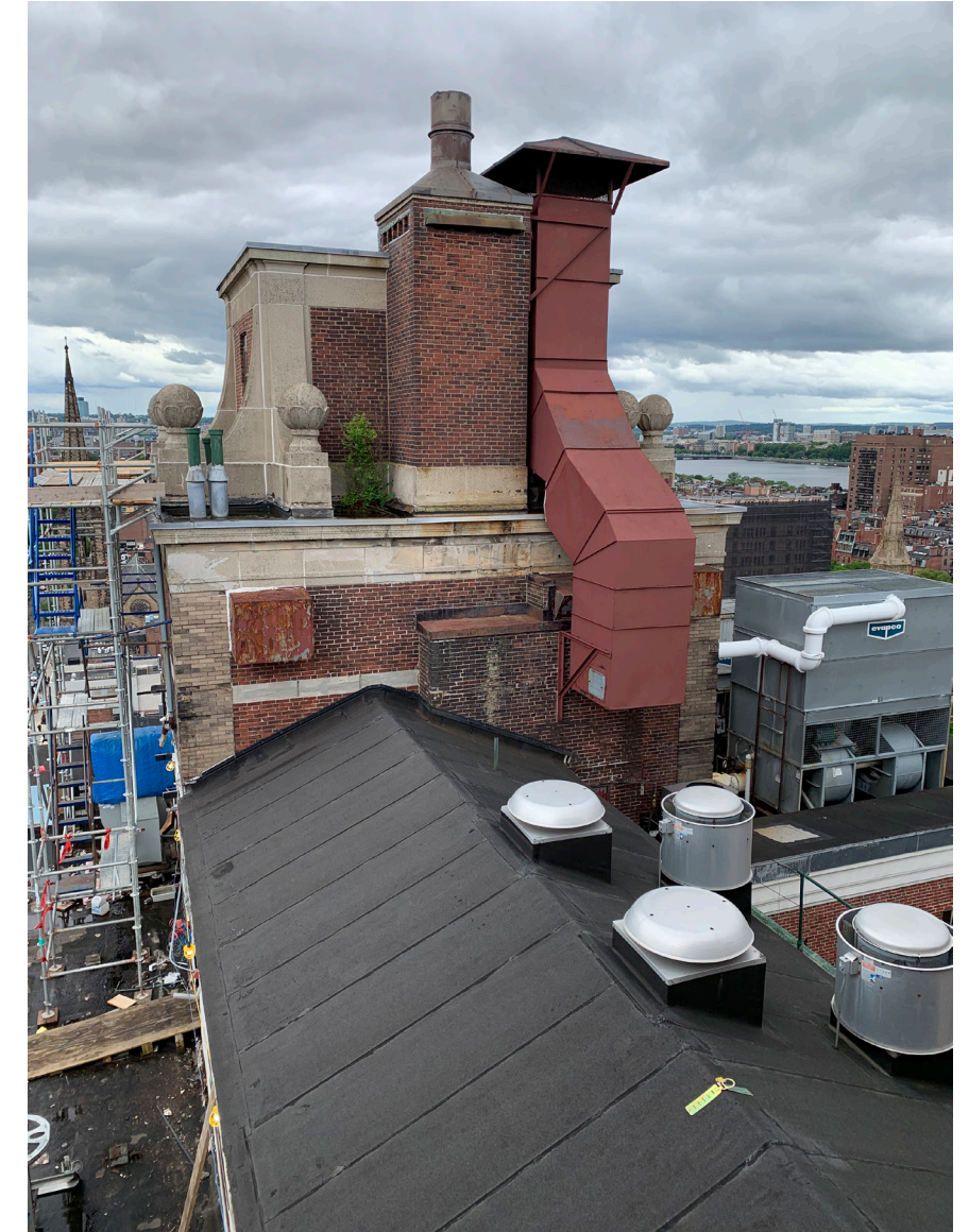
3. REMOVE AND REPLACE ROOFTOP EQUIPMENT
