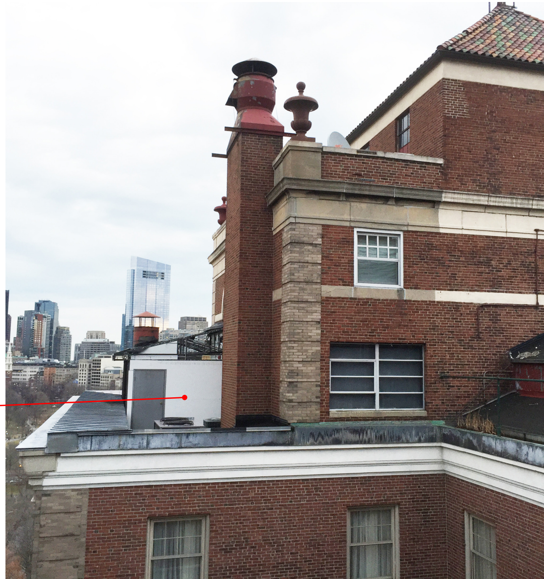
FLR 17 - EXISTING SHED
