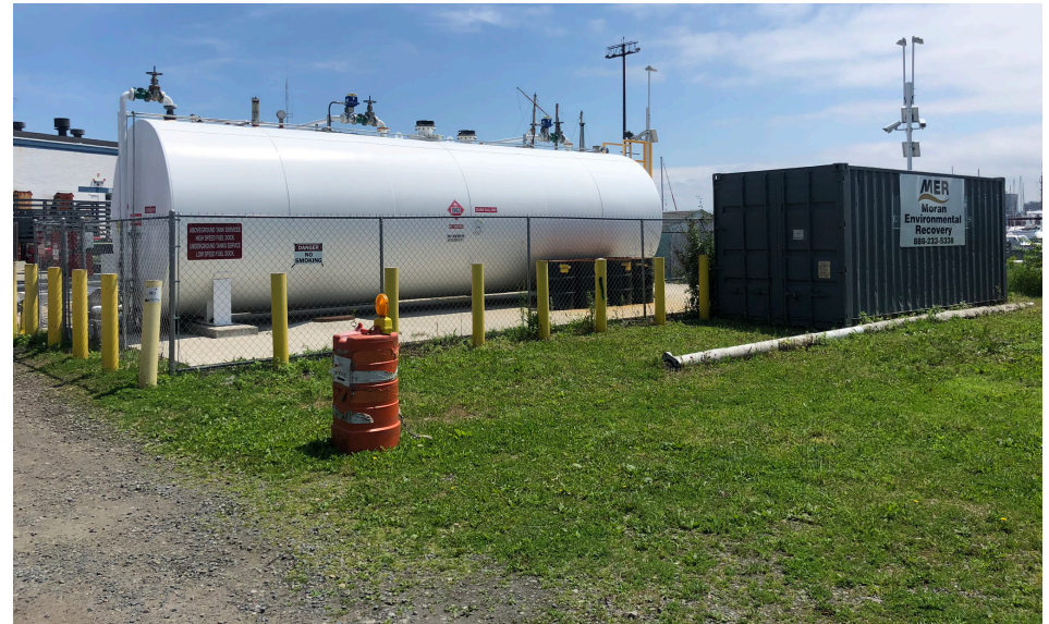
View of Project Site from the northwest.
