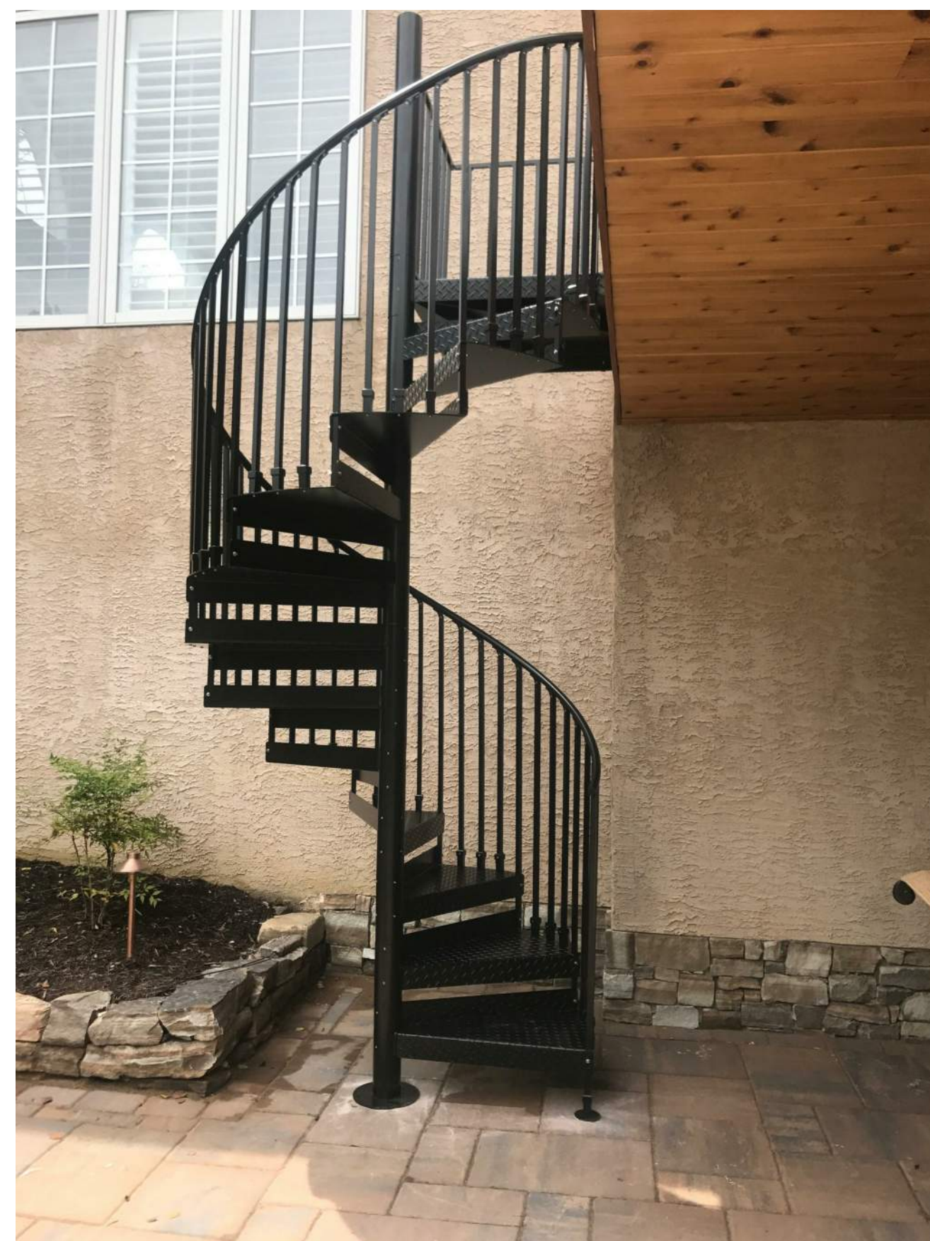
SPIRAL STAIR TO BE USED. BLACK PAINTED METAL TO MATCH EXISTING GUARDRAILS.
