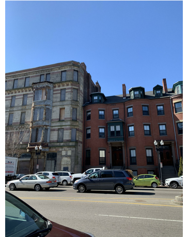
VIEW OF NORTHEAST CORNER
