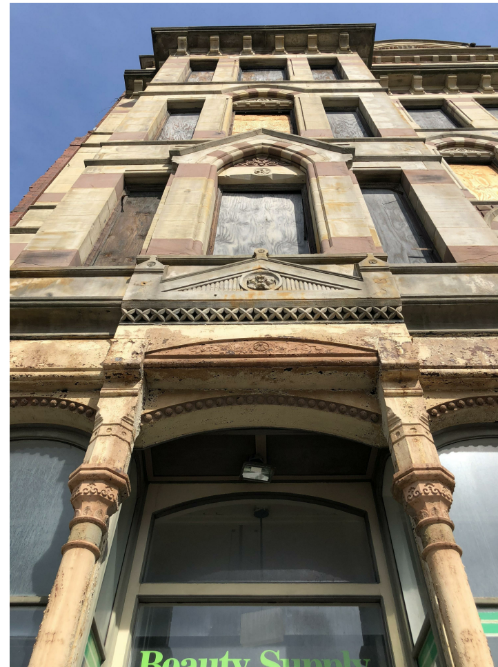
VIEW OF WEST BAY AT SOUTH ELEVATION
