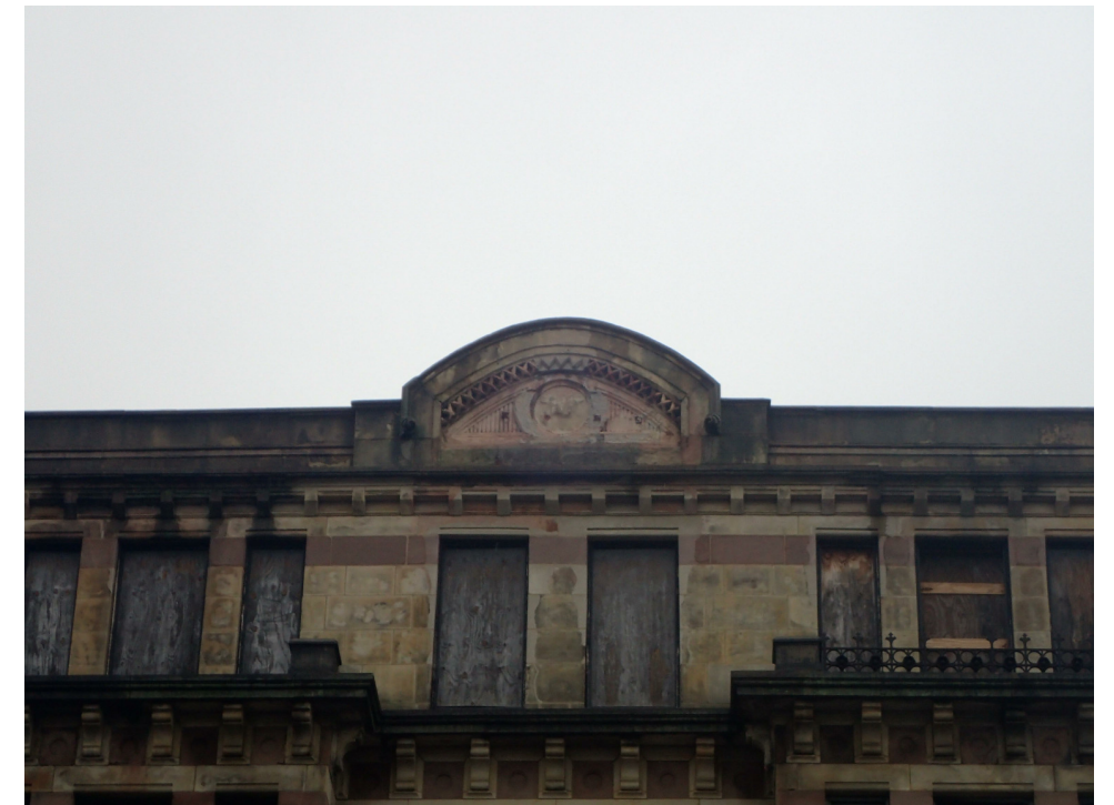
CLOSE UP OF GABLE AND CORNICE AT SOUTH ELEVATION
