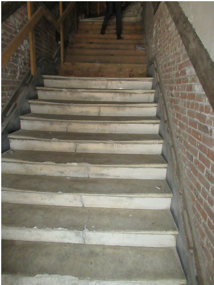
MARBLE ENTRY STAIRS
