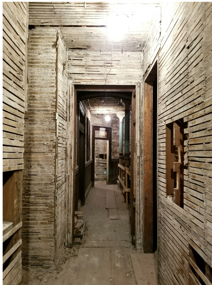
VIEW OF INTERIOR CORRIDOR
