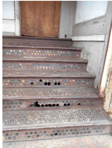
PHOTO 2: EAST ELEVATION, RESTORE CAST IRON STAIRS WITH PRISM LIGHTS
