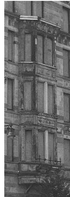
PHOTO 3: EAST ELEVATION, ORIGINAL SHEET METAL BAYS TO BE REPLICATED
