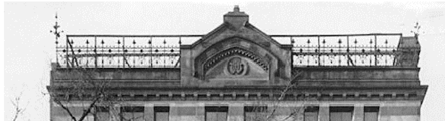
PHOTO 6: ORIGINAL CAST IRON ROOF CRESTING TO BE REPLICATED
