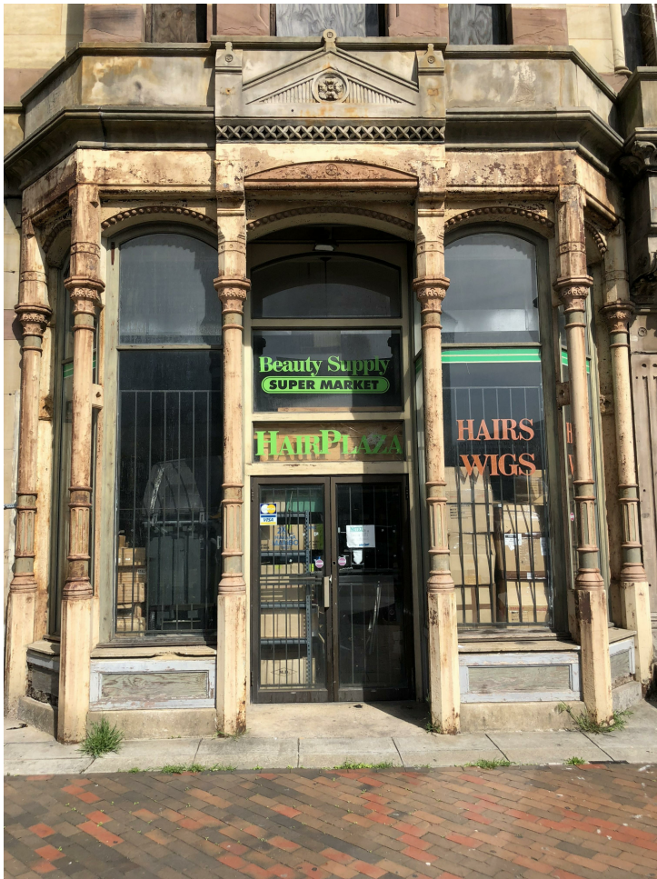
CAST IRON STOREFRONT AT SOUTH ELEVATION
