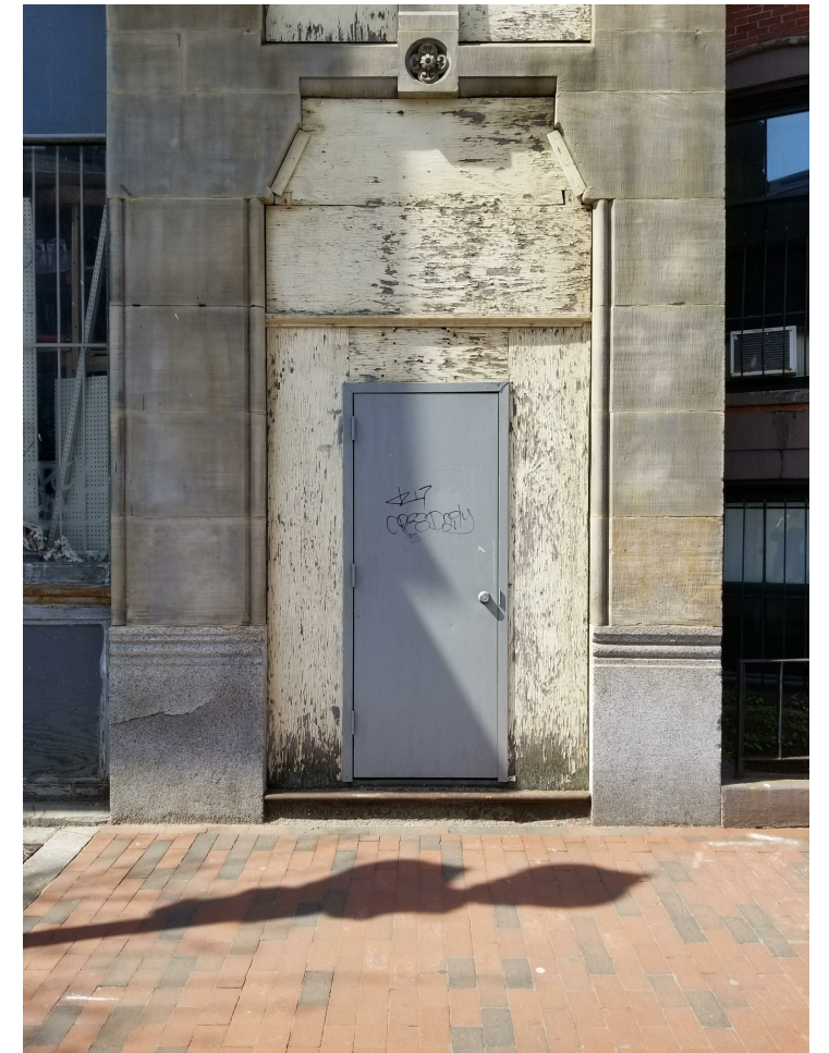
NON-ORIGINAL DOOR AND INFILL AT EAST ELEVATION
