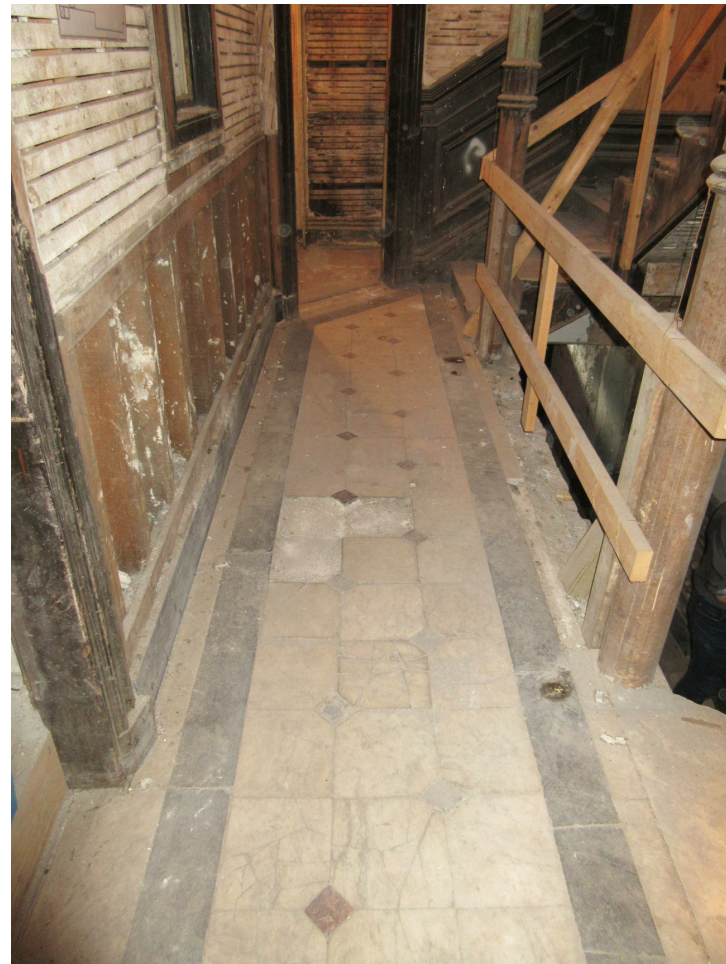
STONE TILE AT LEVEL 2
