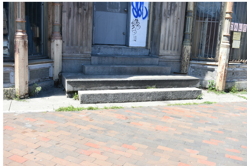
HOTEL ENTRY STEPS AT SOUTH ELEVATION
