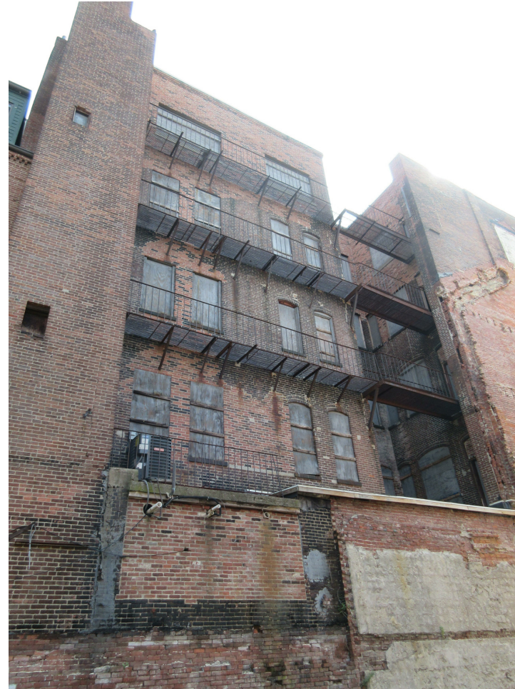
WEST ELEVATION FROM COMET PLACE
