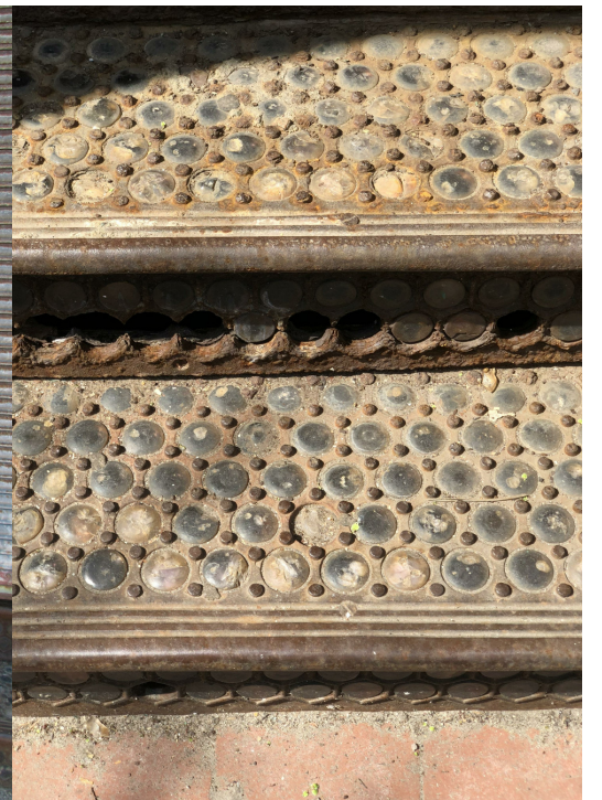
CLOSE-UP OF CAST IRON STAIR
