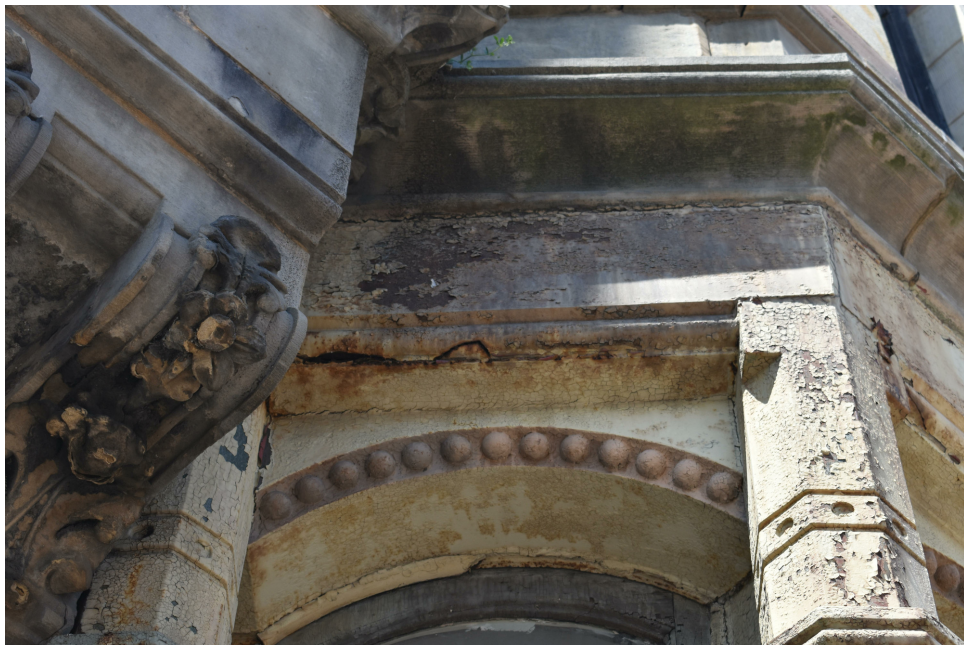
DETAIL AT TOP OF CAST IRON STOREFRONT
