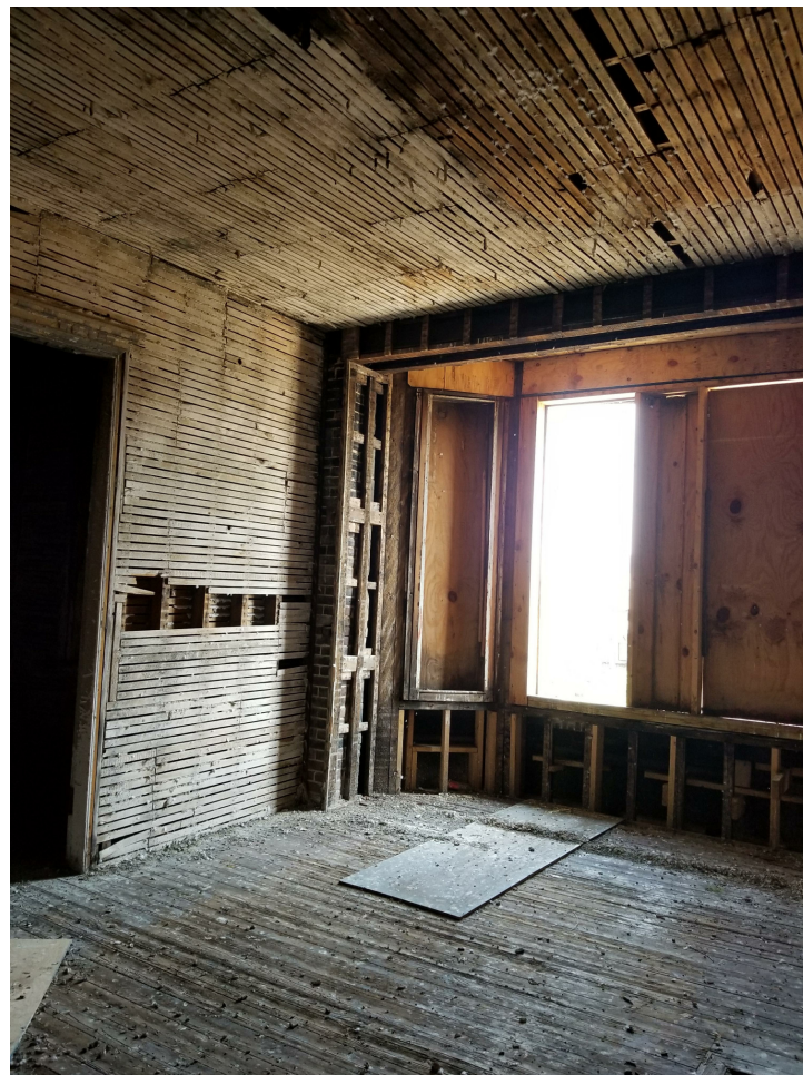
FRAMING AT ORIEL
