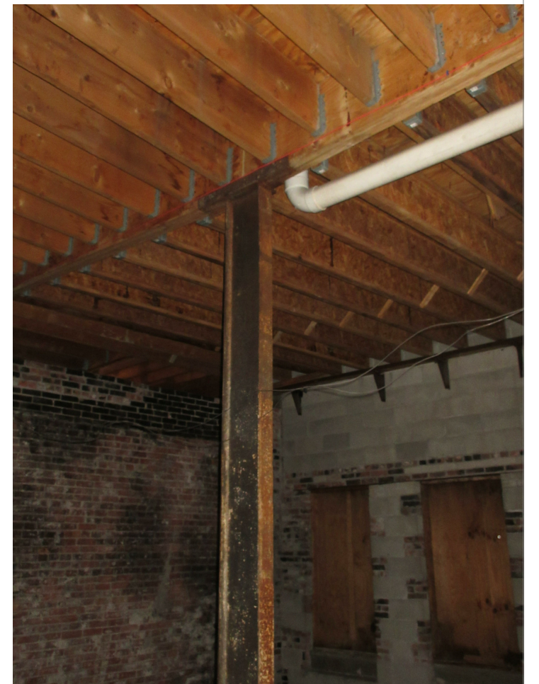
NON-ORIGINAL ROOF FRAMING AND SUPPORT
