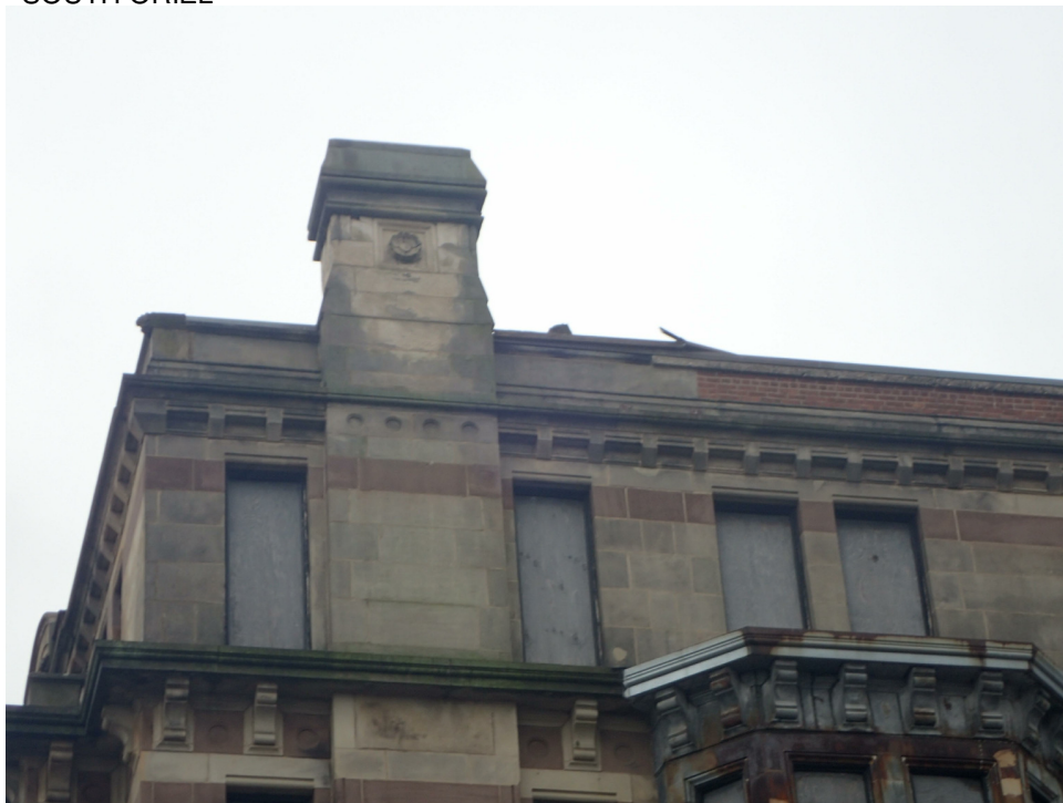
CHIMNEY AND SOUTH ORIEL CORNICE AT EAST ELEVATION
