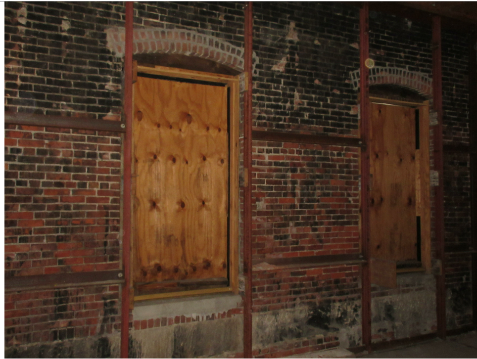
SUPPLEMENTAL BRACING AT EXTERIOR WALL
