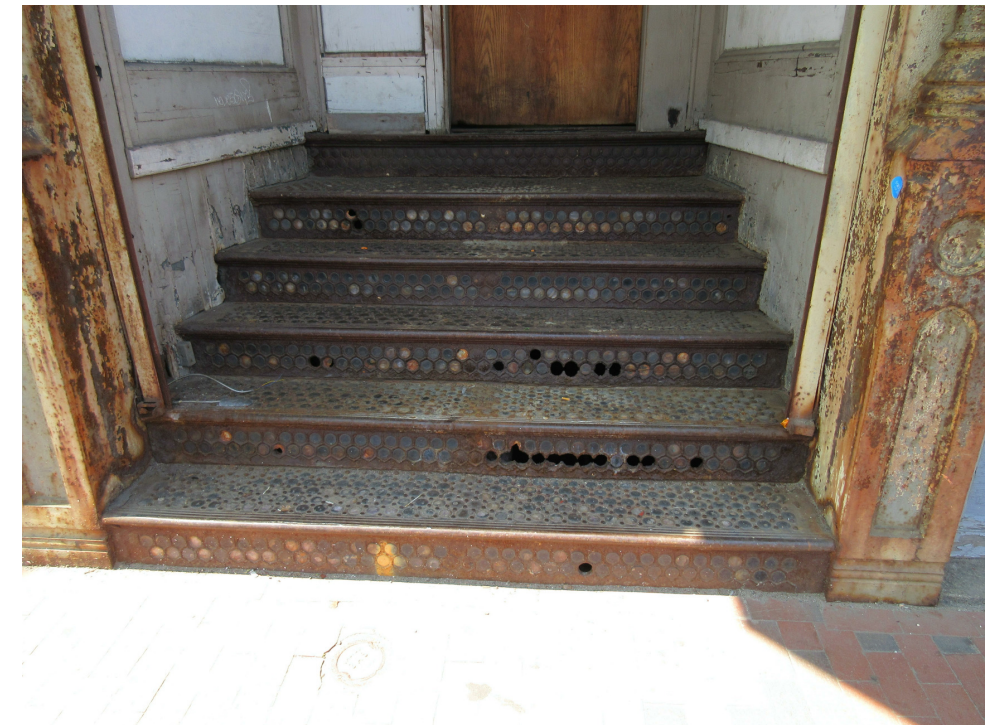
CAST IRON STAIRS WITH PRISM LIGHTS
