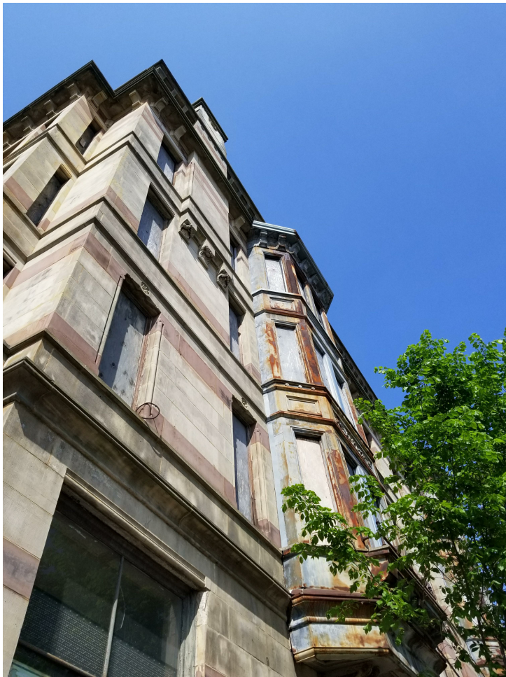
EAST ELEVATION LOOKING UP AT CHIMNEY AND SOUTH ORIEL
