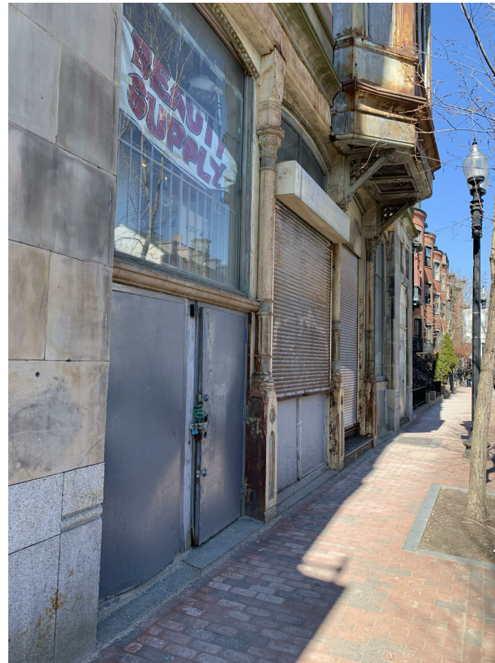
STOREFRONT AND OPENINGS AT EAST ELEVATION
