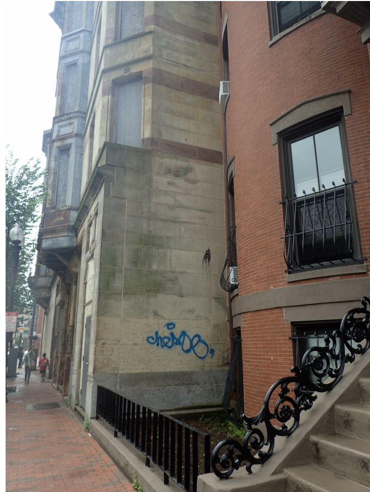
BOTTOM OF NORTH ELEVATION
