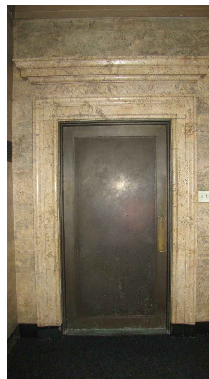
PHOTO 15: CLEARWAY ENTRANCE STONE WALL
