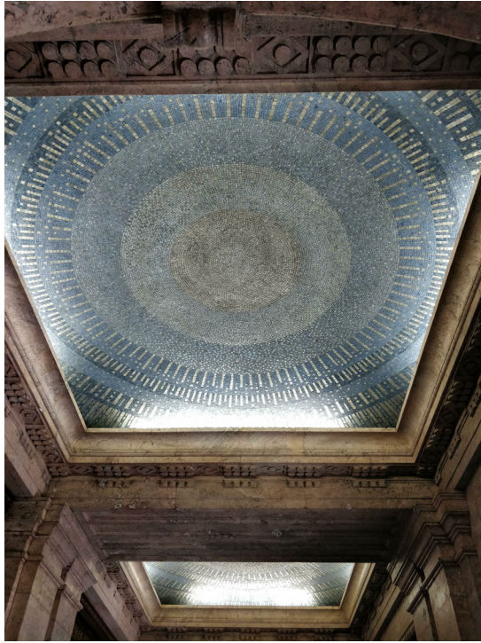
MAIN ENTRY VESTIBULE CEILING
