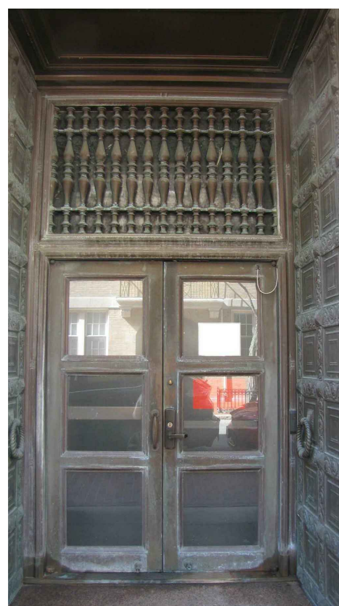
PHOTO 14: VESTIBULE SIDE OF DOOR OPENING
