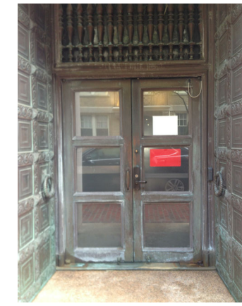
1. STAFF ENTRY CLEARWAY ST.
