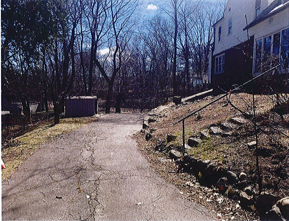
PHOTO NO. 2 – EXISTING BUILDING (REAR)
