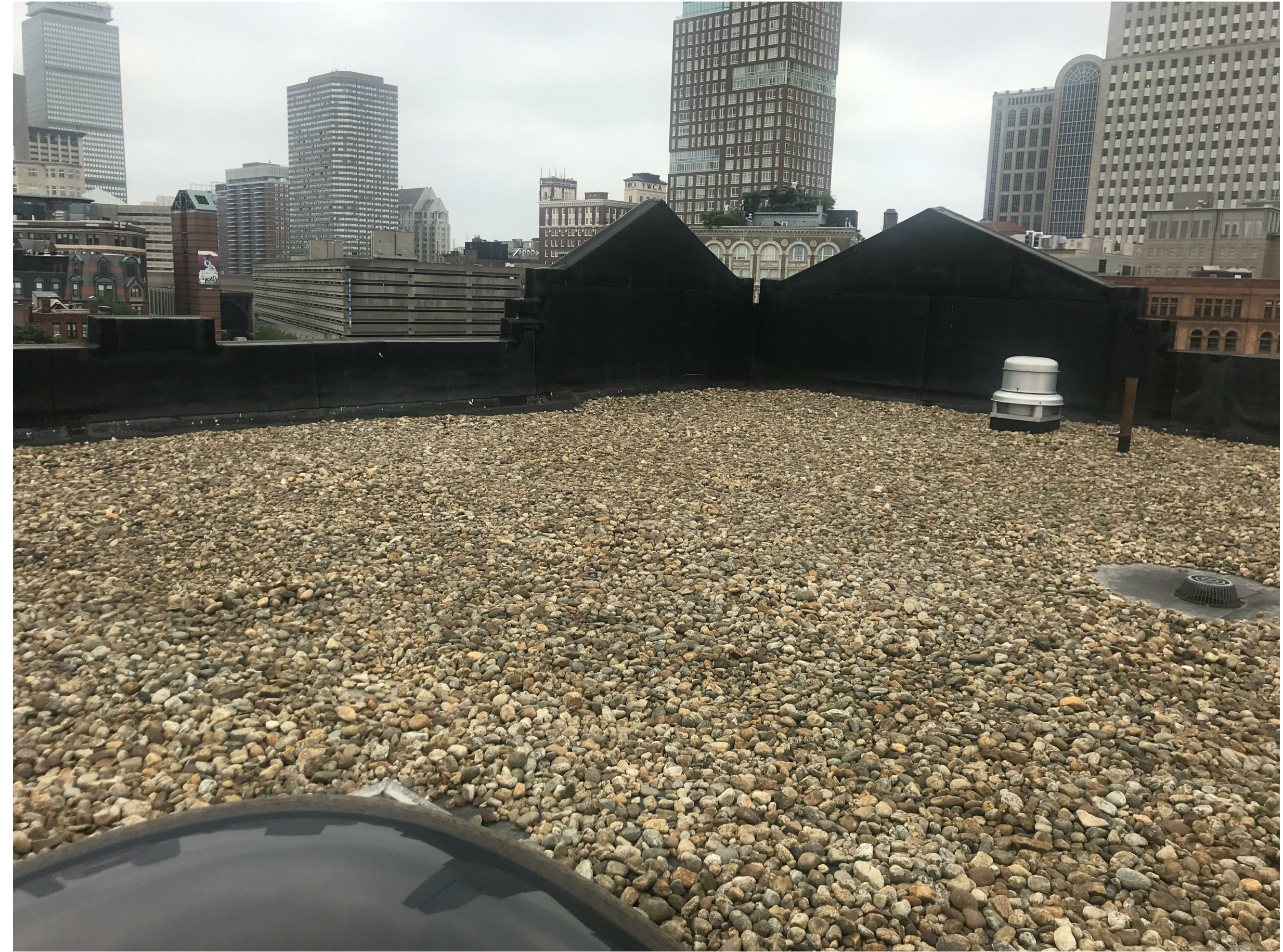
G: VIEW FROM HEAT PLANT LOOKING TOWARDS PROPOSED UNIT
