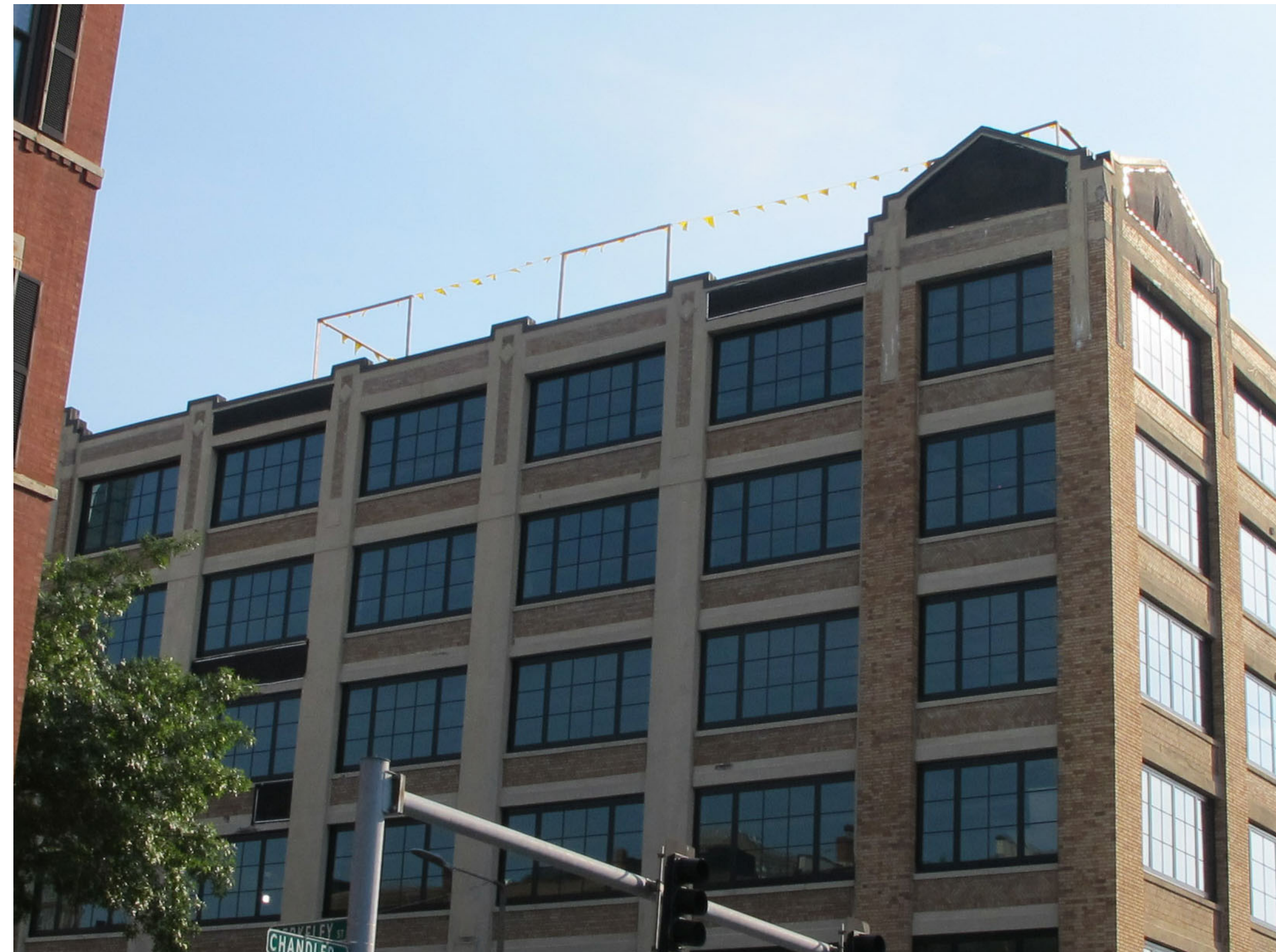
D: VIEW FROM CHANDLER STREET - ENLARGED
