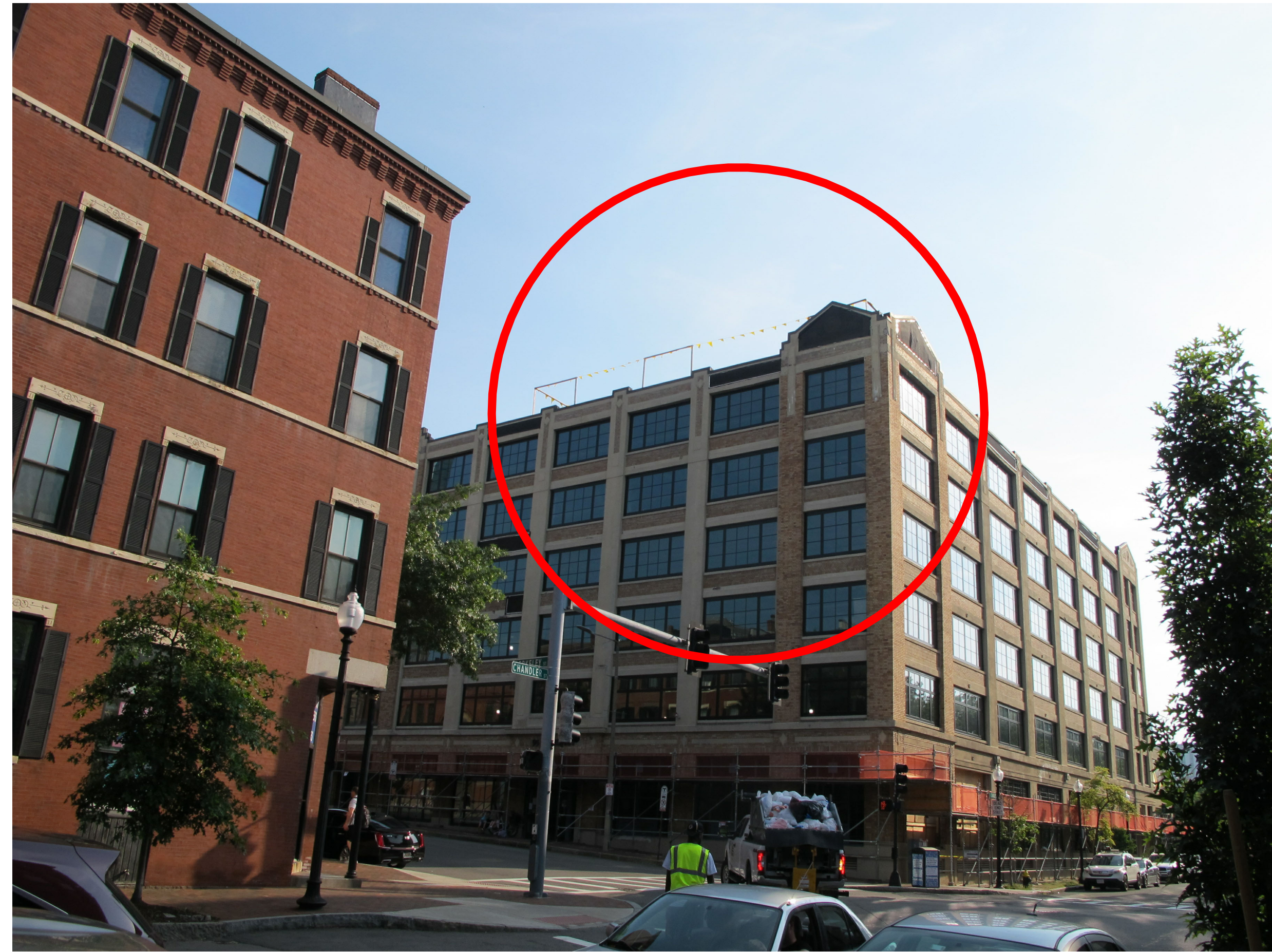
D: VIEW FROM CHANDLER STREET
