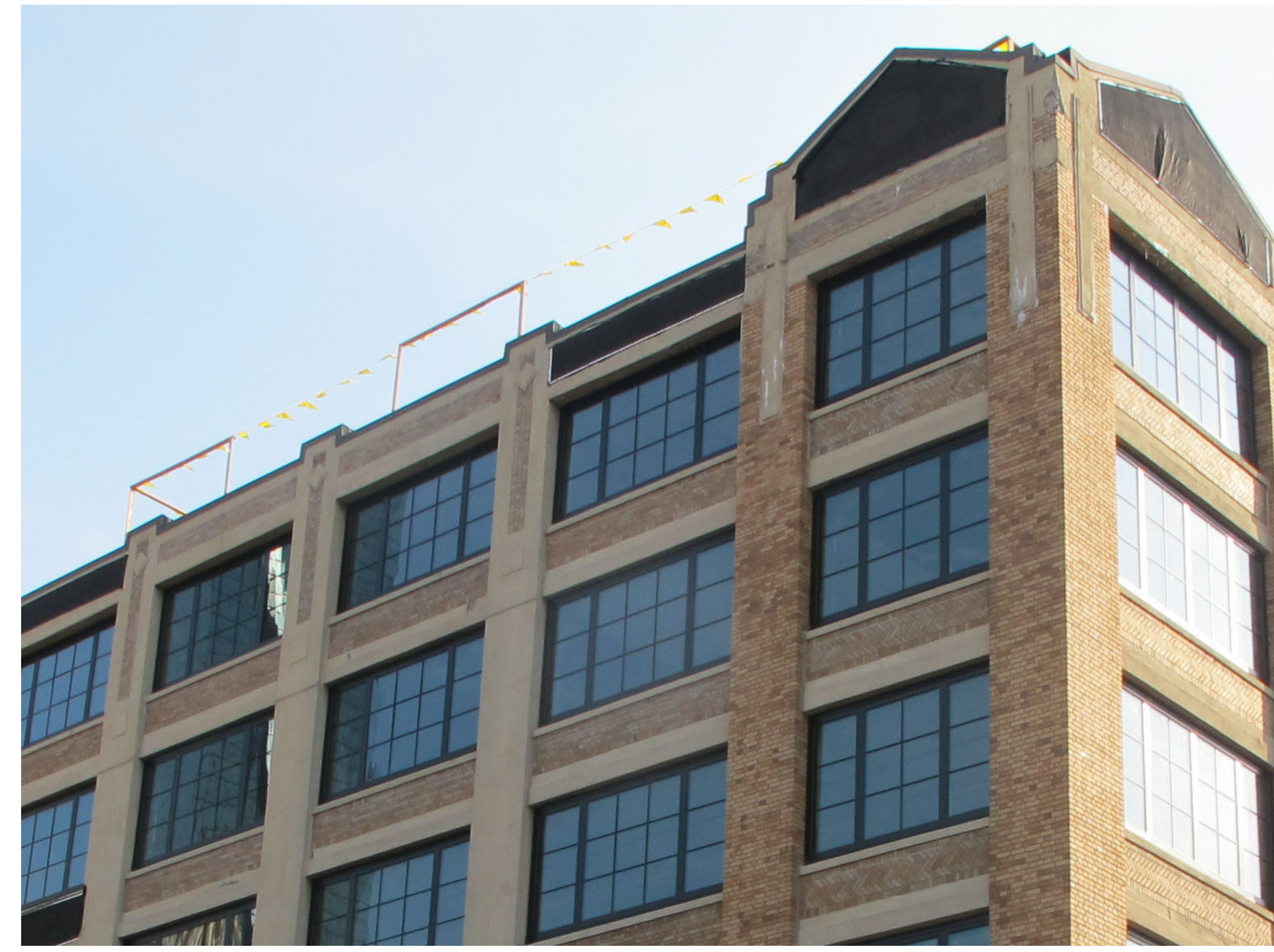
B: VIEW FROM INTERSECTION OF BERKELEY AND CHANDLER ENLARGED
