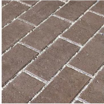
PERMEABLE UNIT PAVERS
