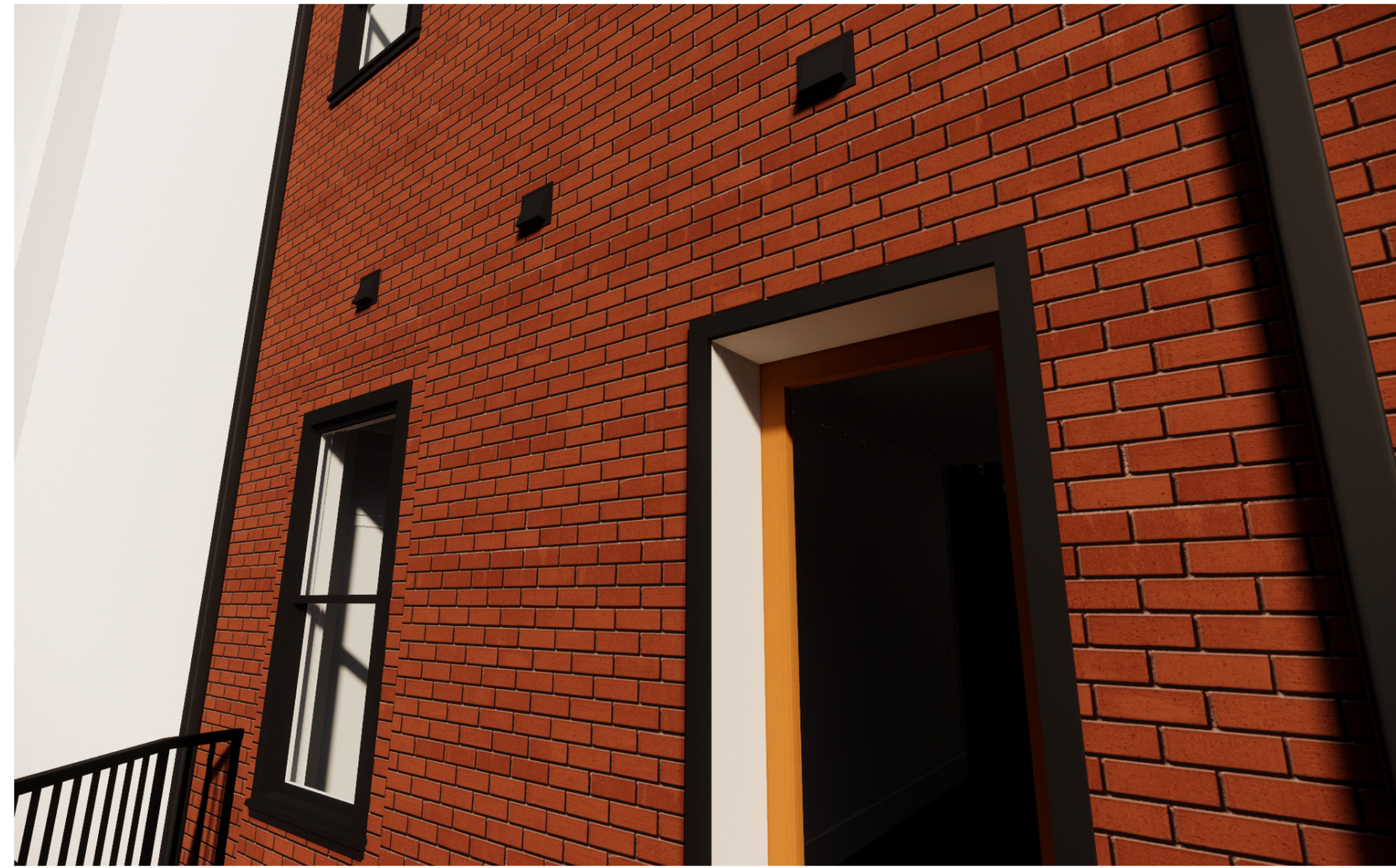
PROPOSED RENDERS OF BACK DECK & PROPOSED ERV / DRYER INTAKE AND EXHAUST VENTS
