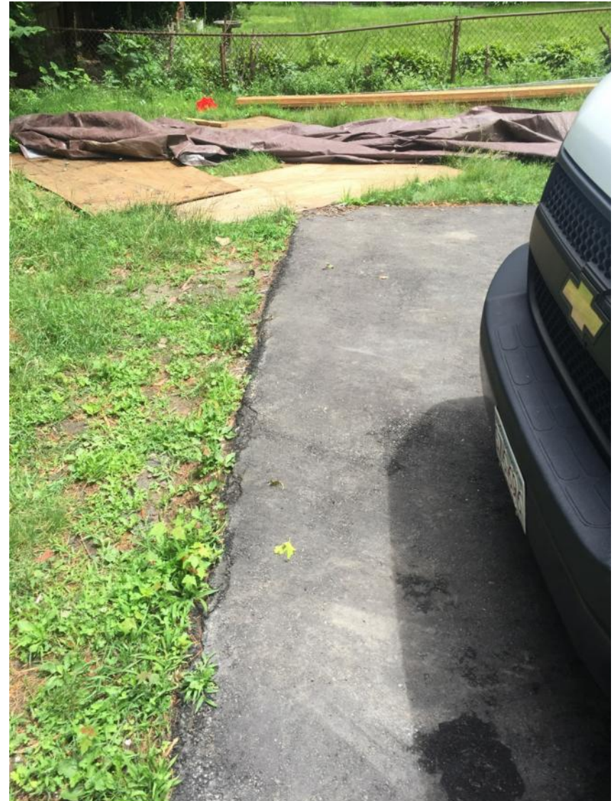
Photo 6. View of driveway in rear yard. Driveway installed at existing grade.
