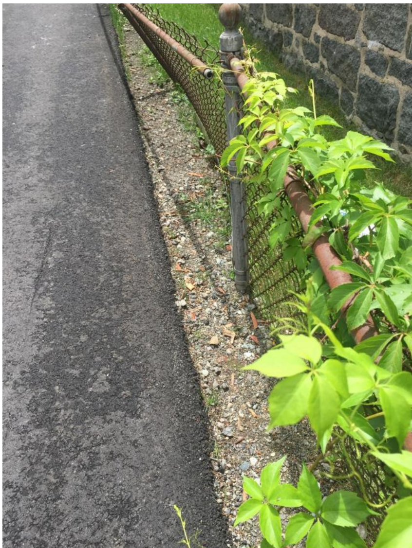
Photo 7. View of driveway in side yard. Driveway installed at existing grade.
