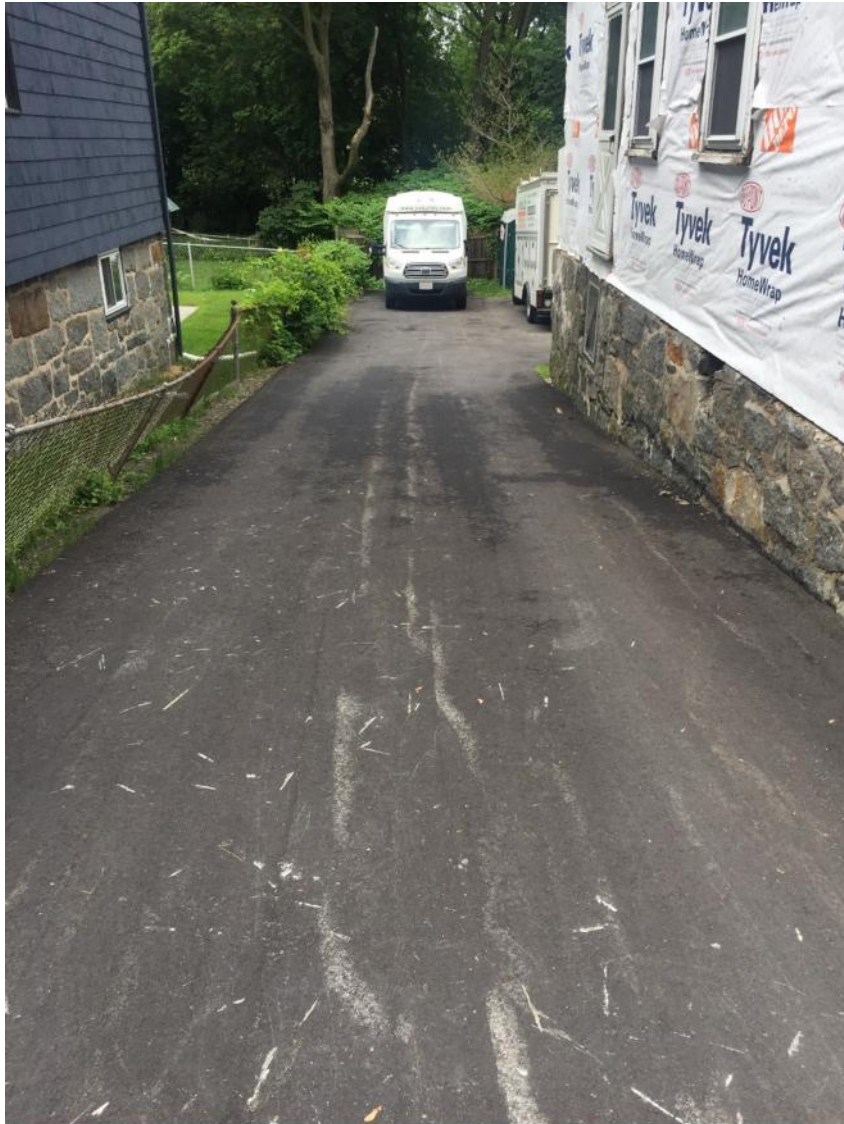
Photo 3. View of driveway extending along side and rear yard.
