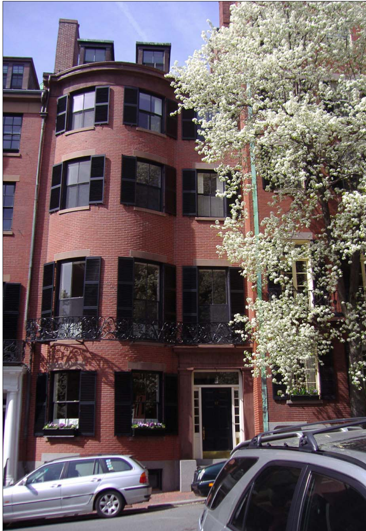
1 EXISTING VIEW 1 - VISIBLE FROM PINCKNEY STREET
