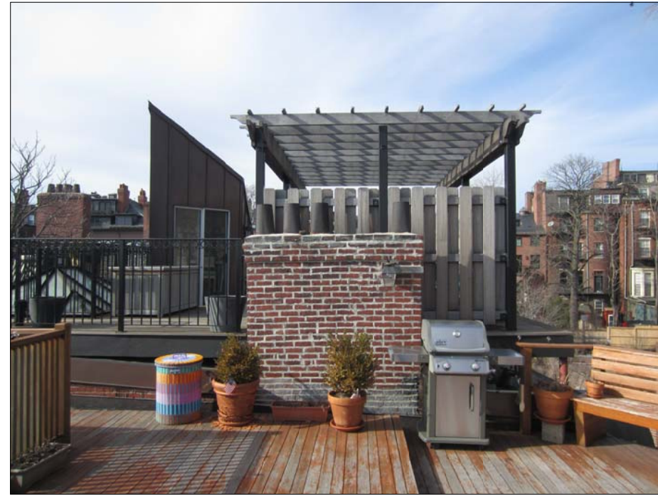
EXIST DECK WITH NEIGHBORS DECK BEHIND CHIMNEY, LOOKING NORTH
