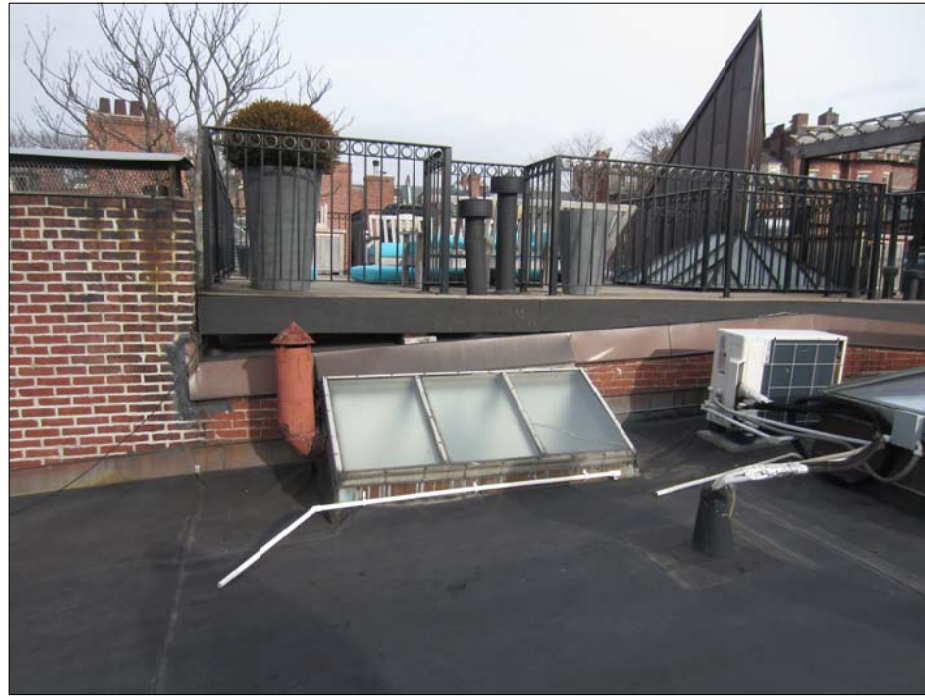
EXIST SKYLIGHT TO BE REMOVED, LOOKING NORTH
