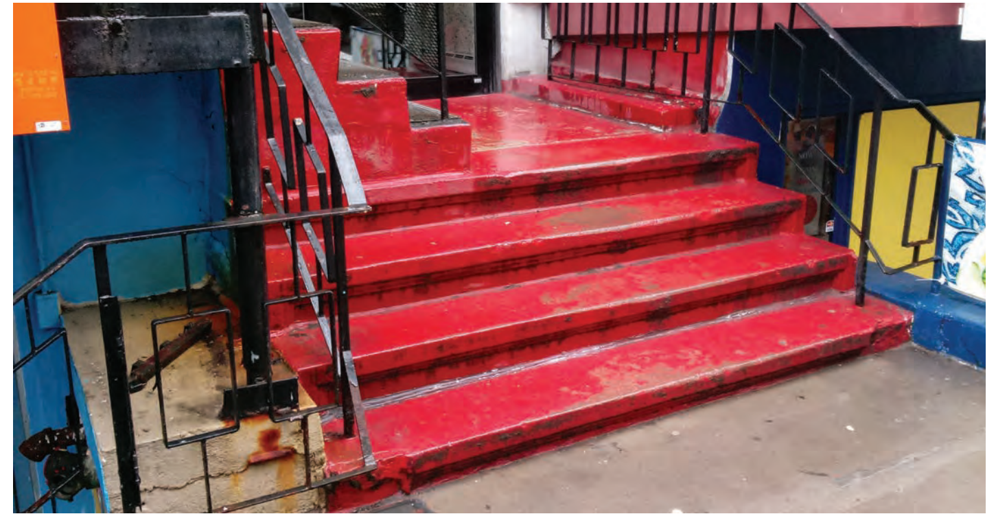
Entry Stair at 829
