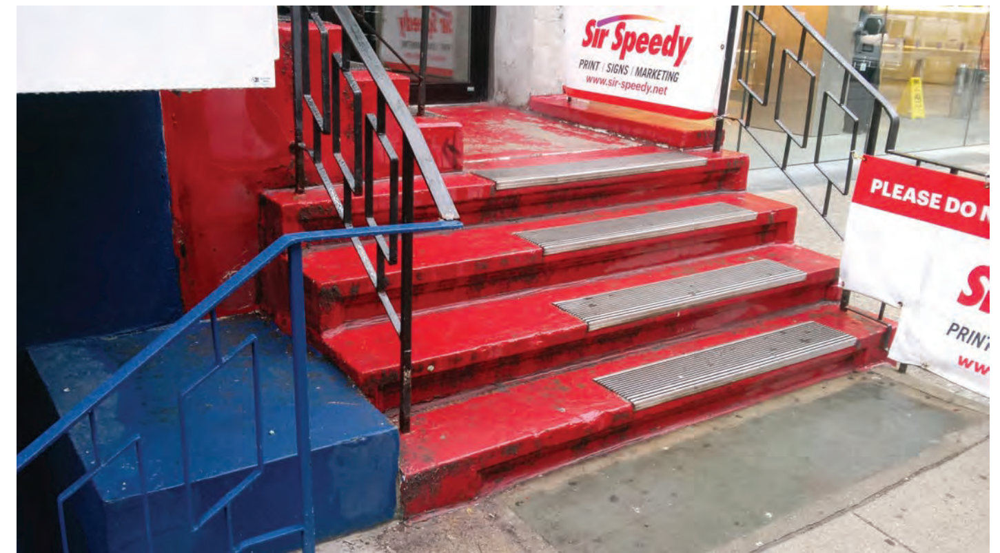
Entry Stair at 827
