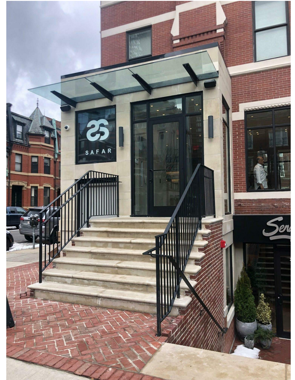
235 NEWBURY STREET - SAFAR SALON ENTRY (NEWBURY & FAIRFIELD)
