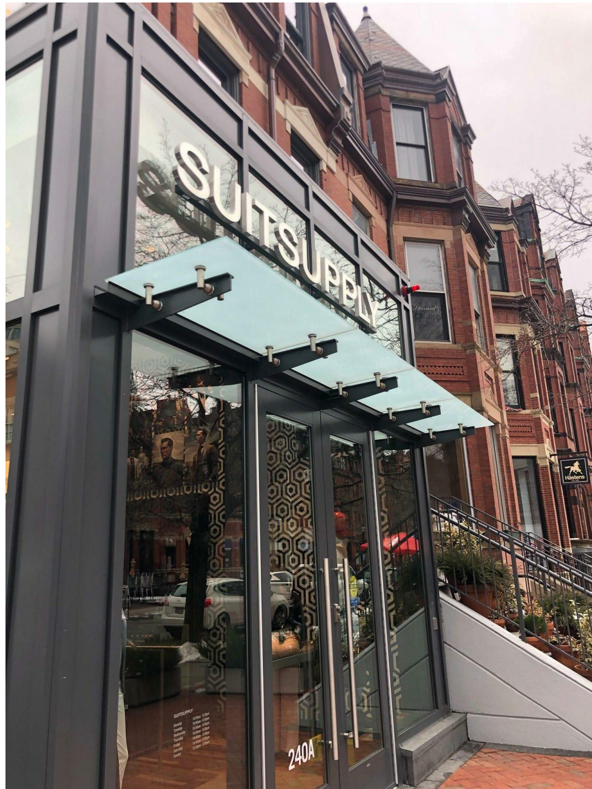
MODERN GLASS & STEEL CANOPY - LOCATED AT 240 NEWBURY STREET
