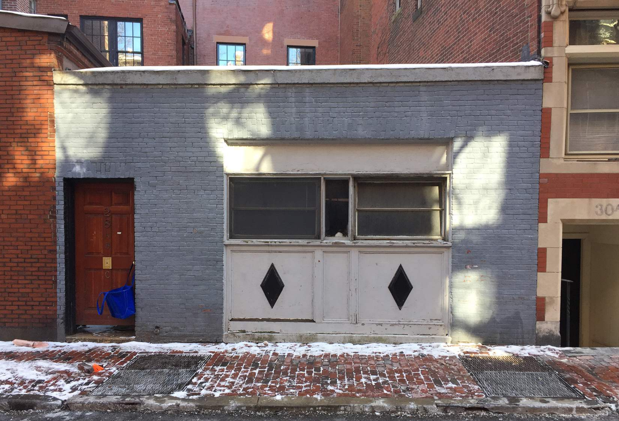
28 PINCKNEY STREET [IMAGE 1] EXISTING EXTERIOR PHOTOGRAPH
