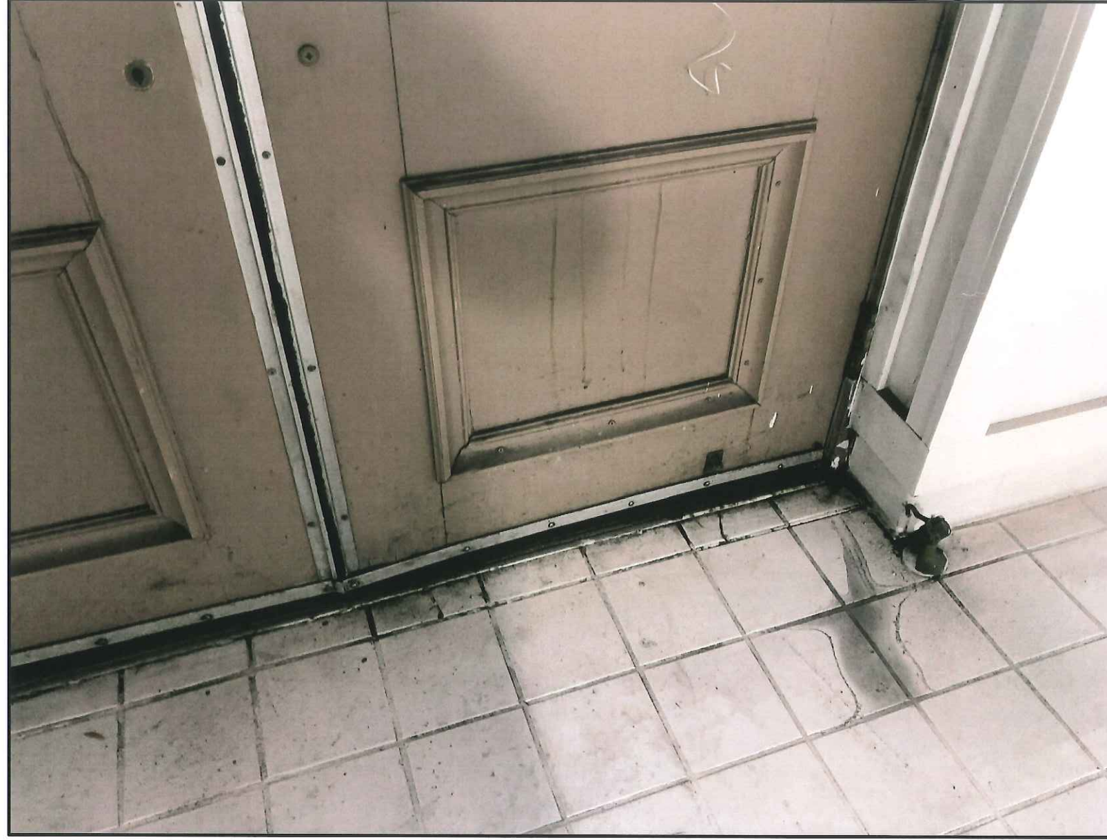
① EXTERIOR DOOR- INTERIOR IMAGE
