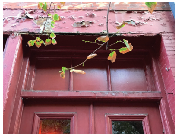
WOOD PANELS IN TRANSOM
