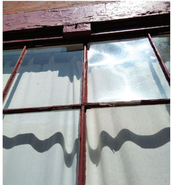
FIRST FLOOR FIXED WINDOW MUNTINS
