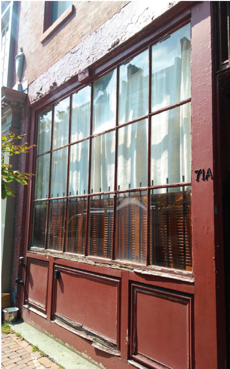
FIRST FLOOR FIXED WINDOW SASH & STEEL BEAM
