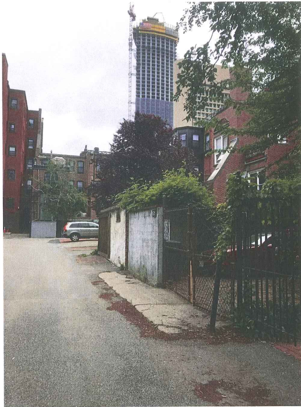
REAR ALLEY FACING NORTH
