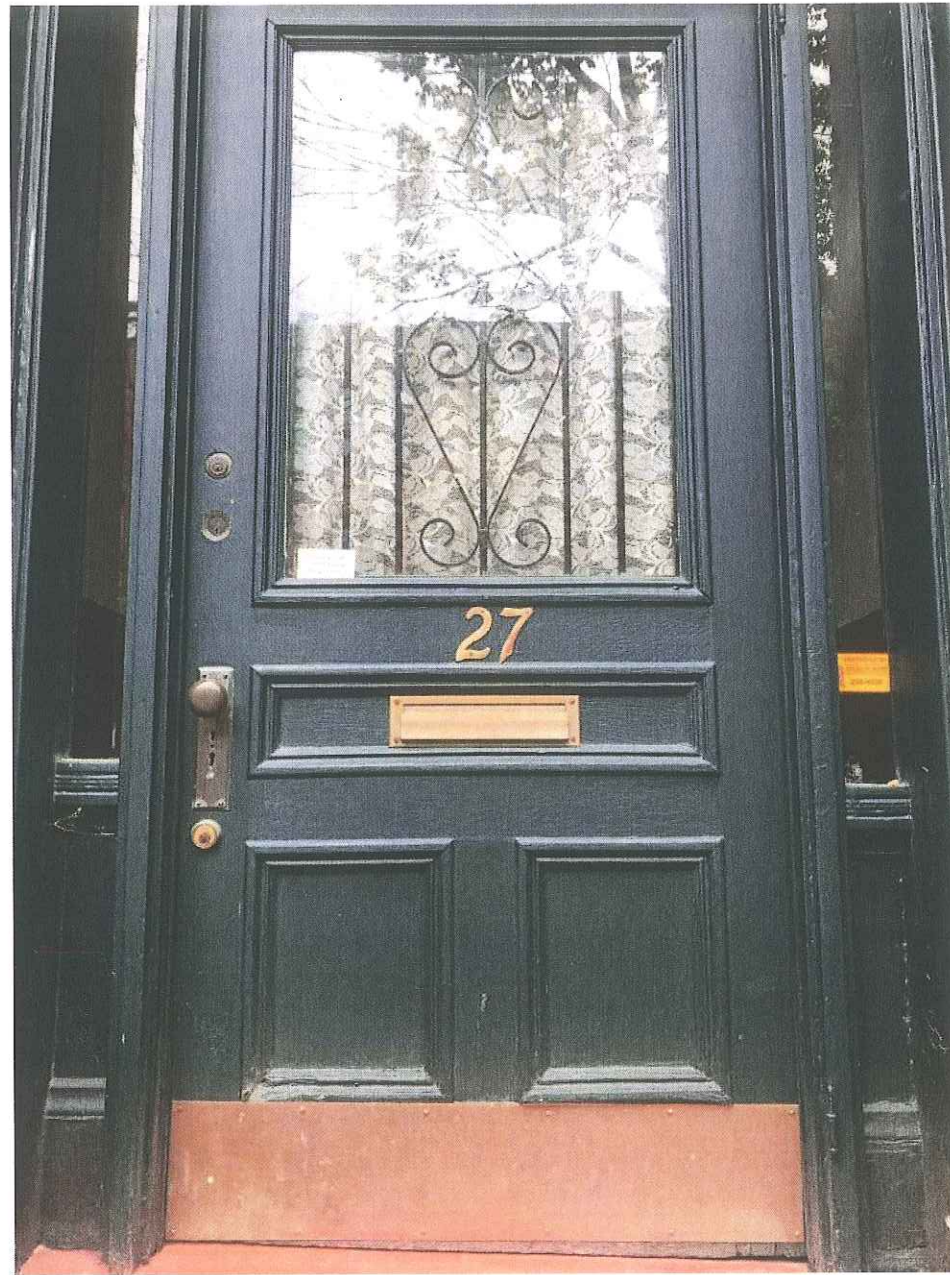
EXISTING FRONT DOOR
