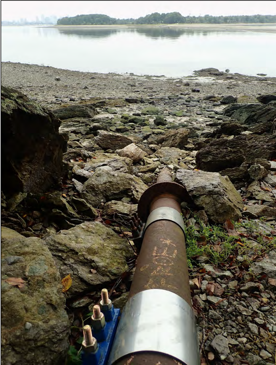
View north (from Mainland Quincy) showing exposed water main.
