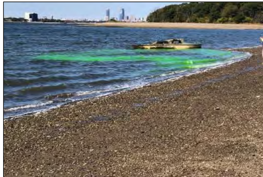
Location of water main break via dye test results (looking northwest).
