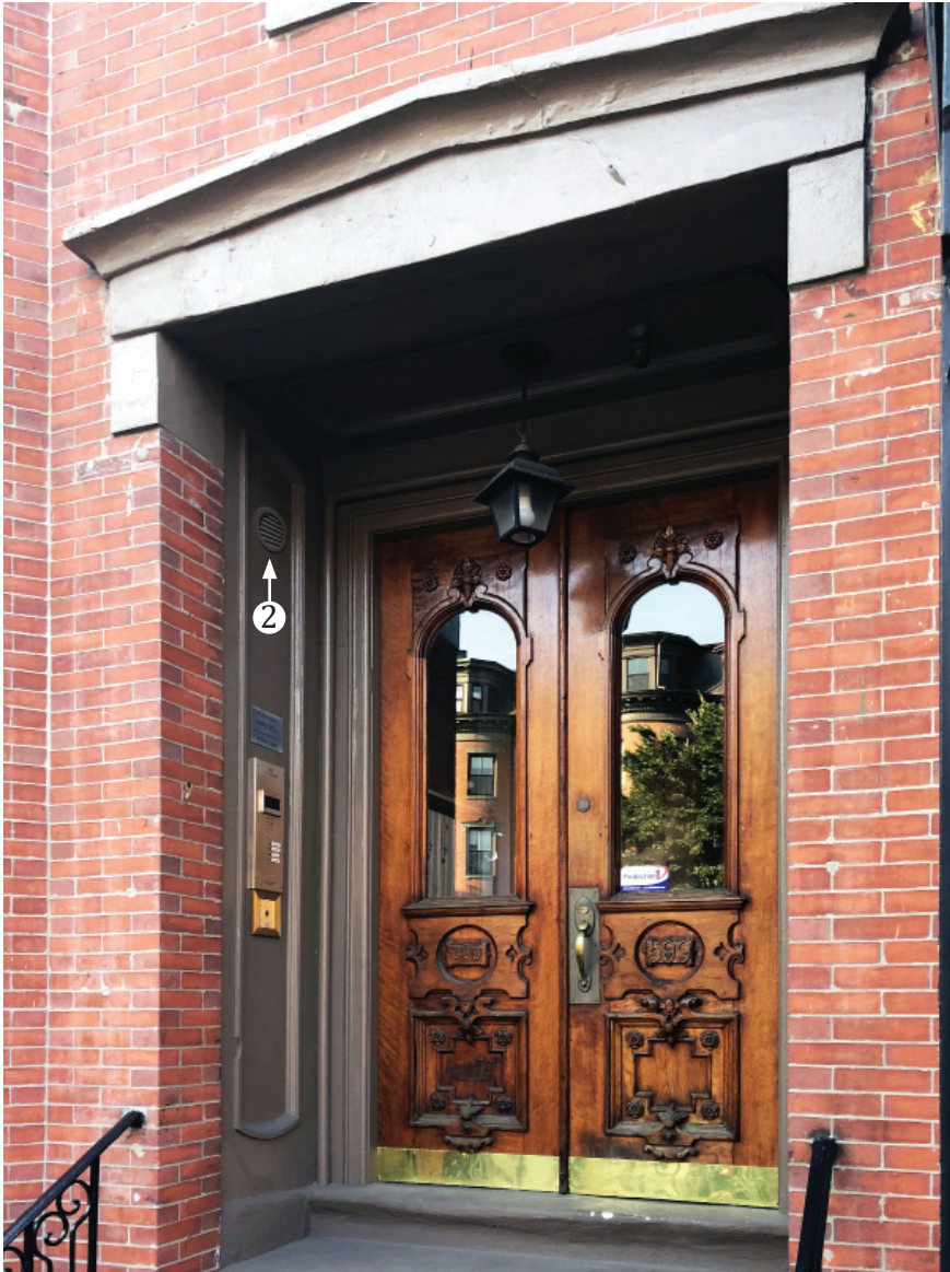
View of proposed ventilation port at Entry.
