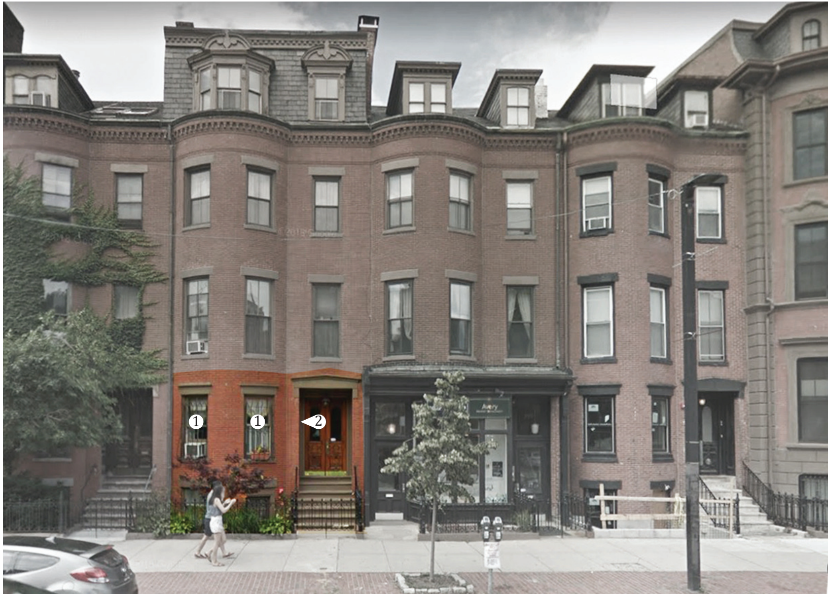
View of existing conditions, 599 Tremont Street. Affected area shown in color.
