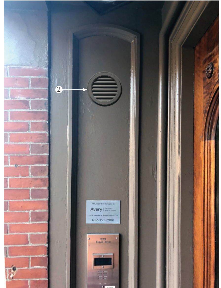
Detail of proposed round ventilation port.
