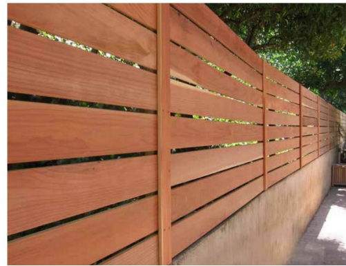
Horizontal cedar fencing
