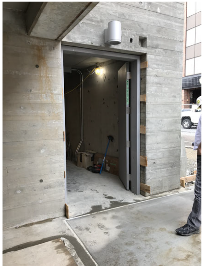
Parks maintenance room Interiors work
