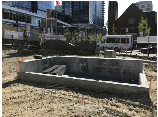
Foundations and forms for wooden seating
