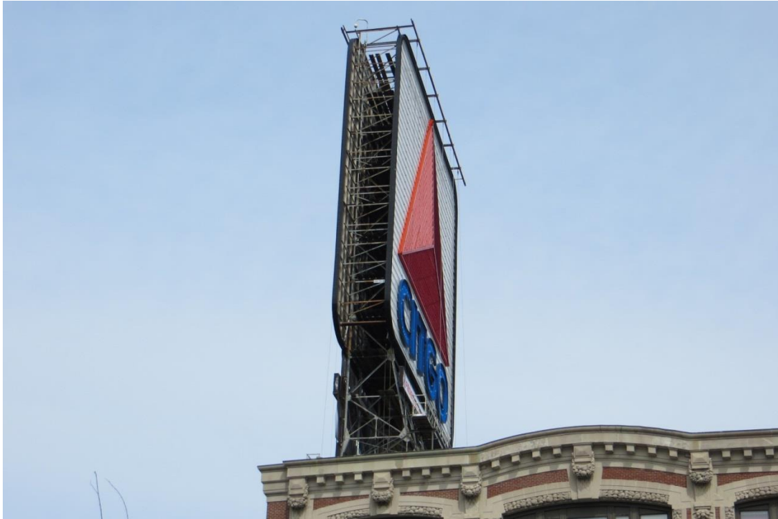
FIGURE 2.3.3 Close-up of the east face of the Citgo sign and supporting steel truss. Photo by Dayl Cohen
