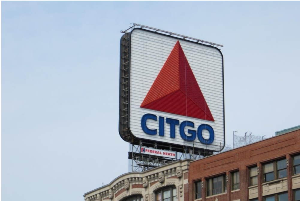
FIGURE 2.3.1 Close-up view from Commonwealth Avenue of east face of the Citgo sign on the roof of 660 Beacon Street. Photo by Dayl Cohen
