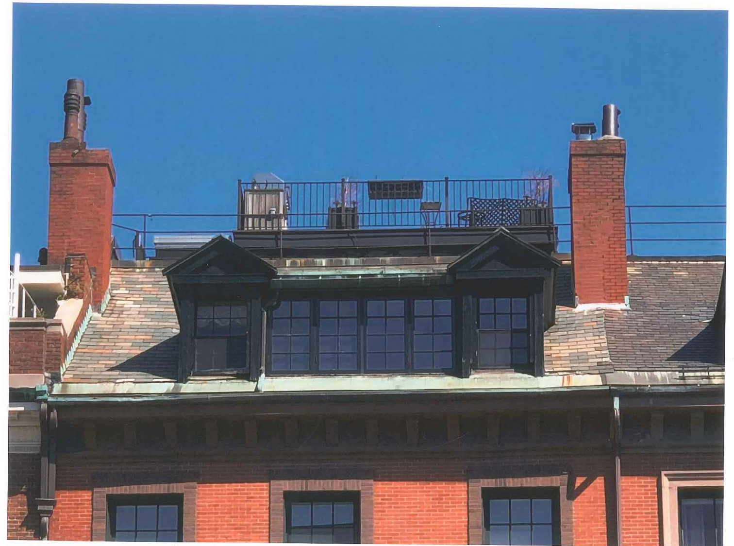
ZOOM-IN VIEW OF THE ROOF DECK FROM THE BOSTON PUBLIC GARDEN PHOTO TAKEN IN 2018
