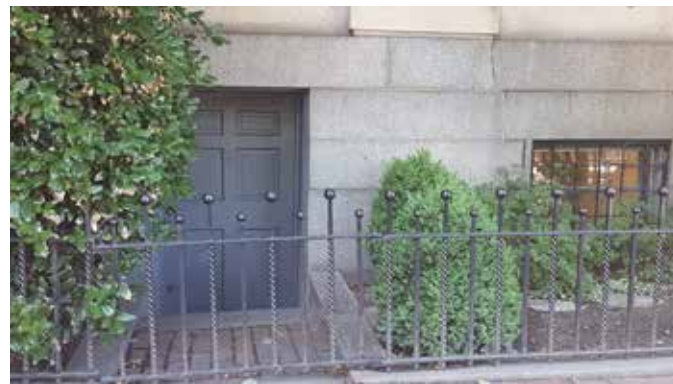
Existing Basement Entry
