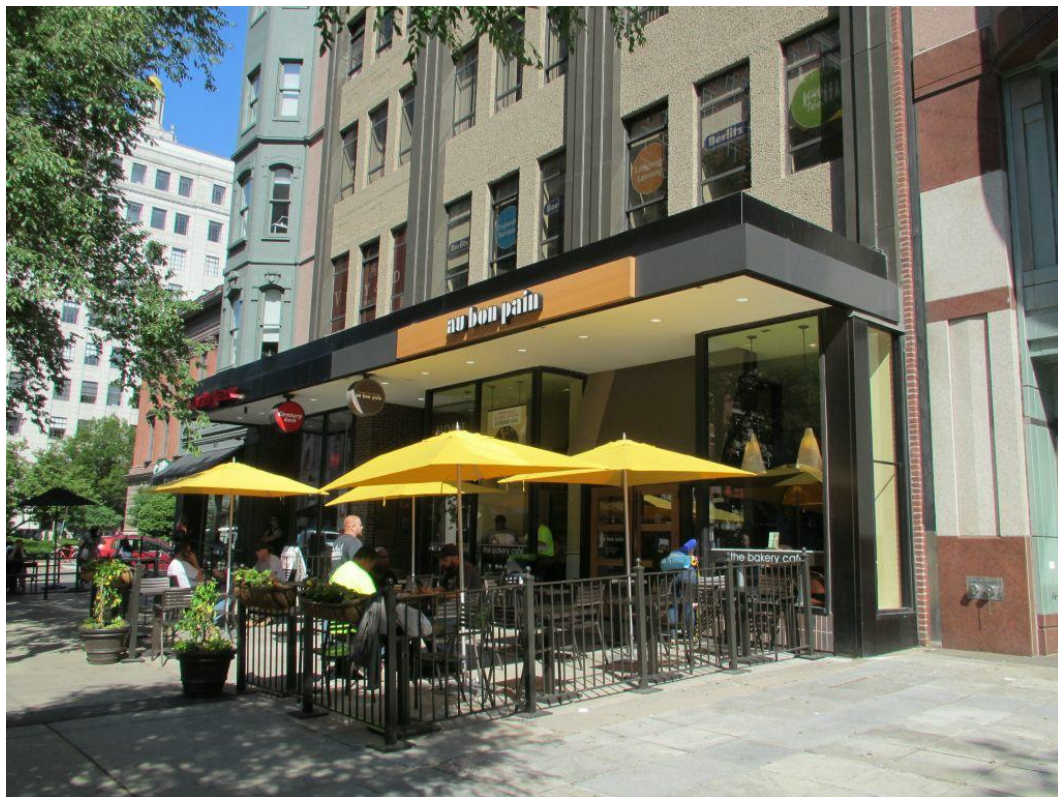
EXISTING EXTERIOR PHOTOS
