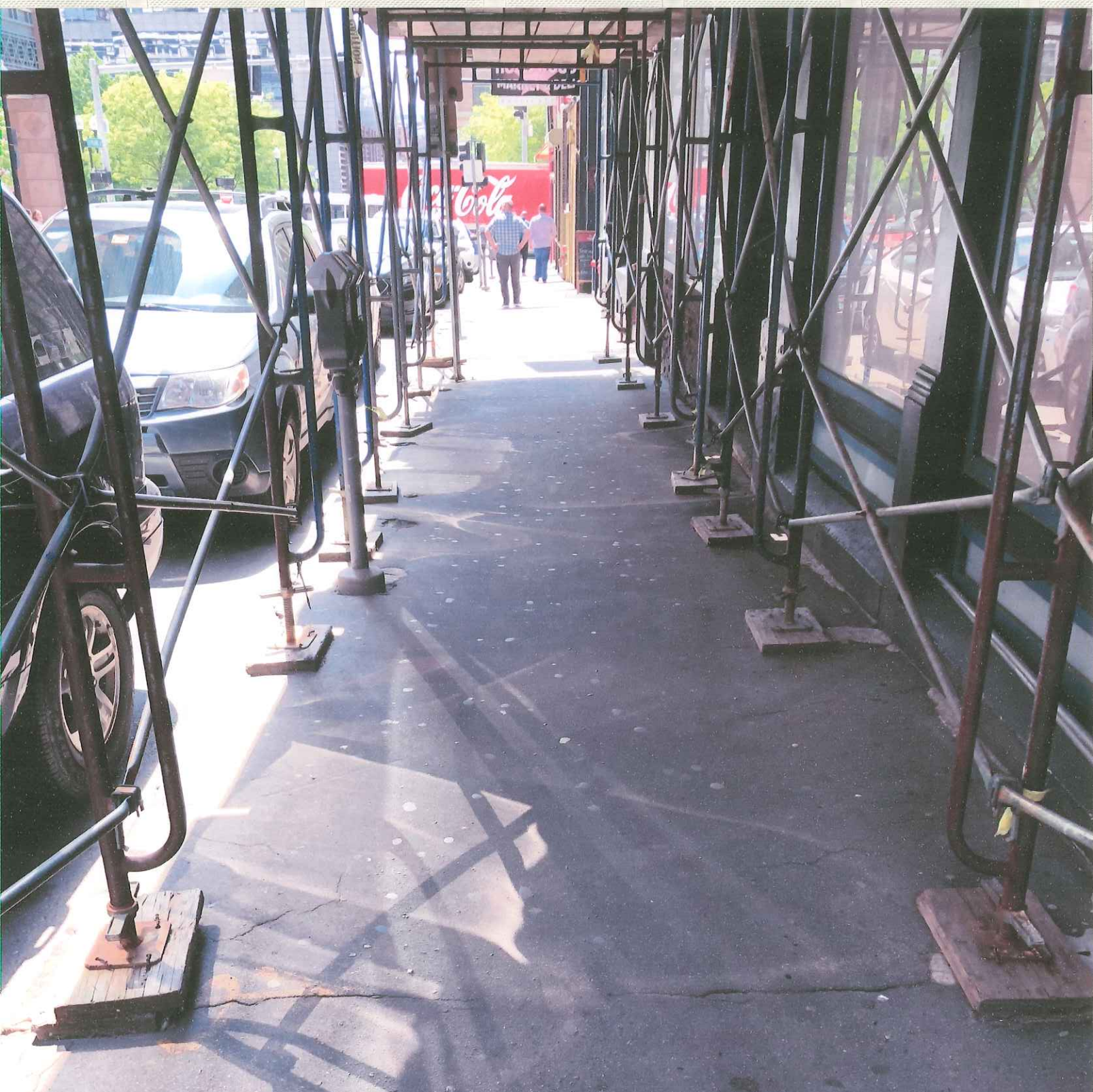
Sidewalk of 115-123 Pearl Street Looking towards Atlantic Avenue
