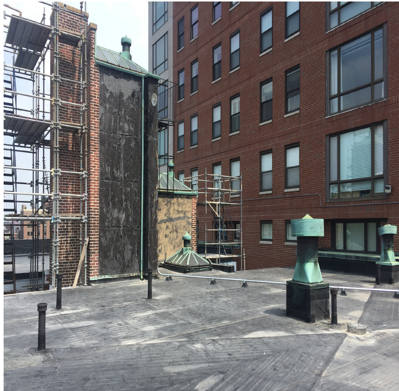
1. NORTHEAST ROOF TOP VIEW
