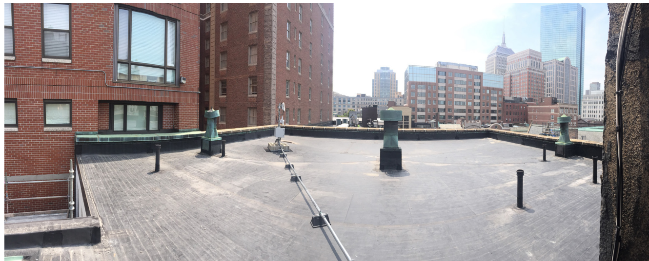
6. SOUTHEAST ROOF TOP VIEW
