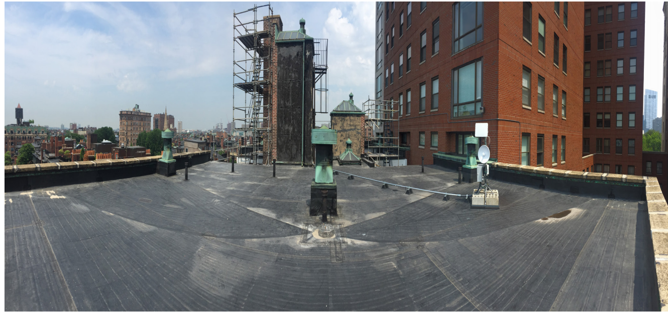
5. NORTH ROOF TOP VIEW
