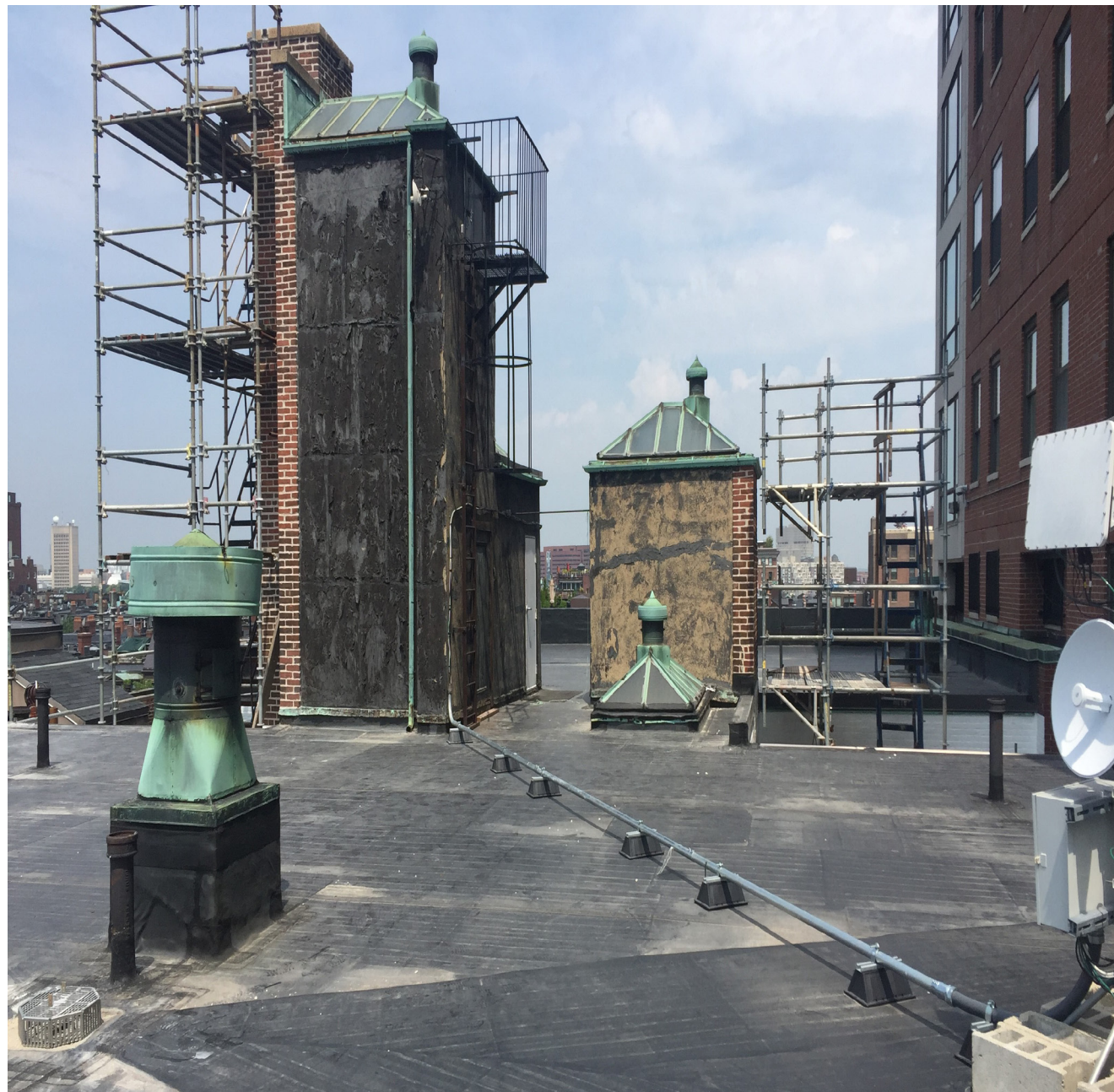
3. NORTHWEST ROOF TOP VIEW
