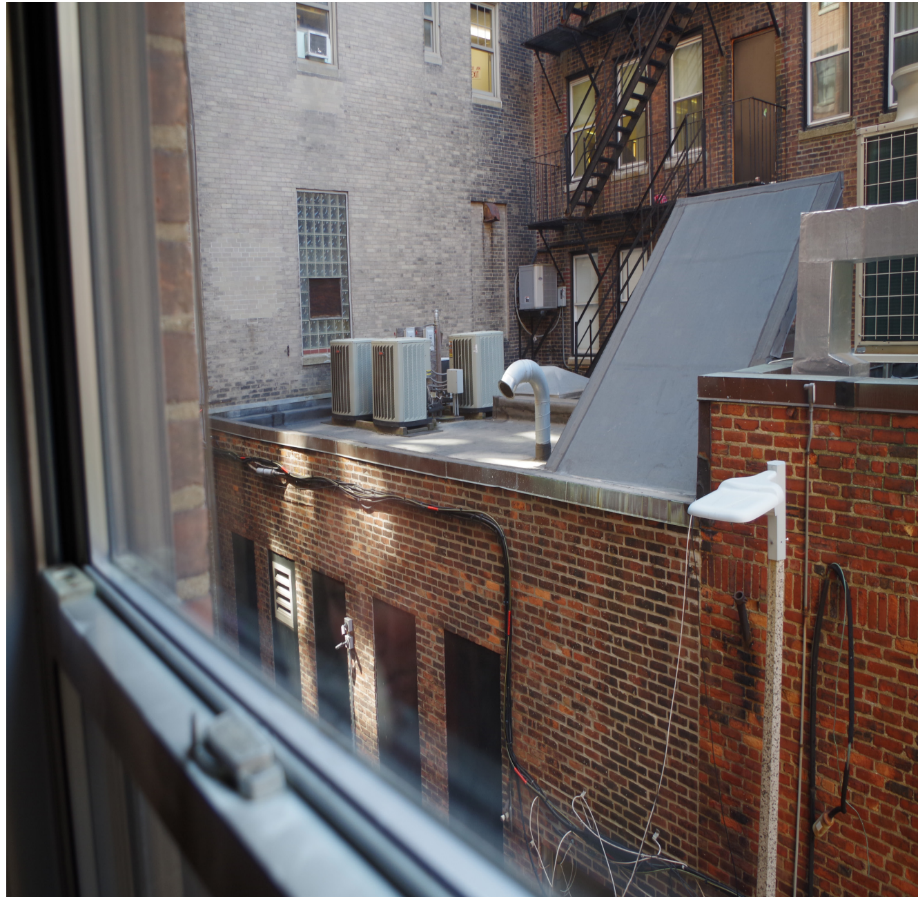
VIEW FROM 2ND FLOOR OF 12 COMMONWEALTH AVE. ACROSS ALLEY
