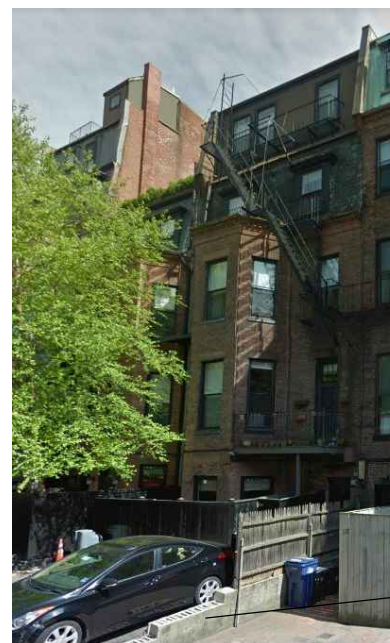
115 MARLBOROUGH STREET - ALLEY
