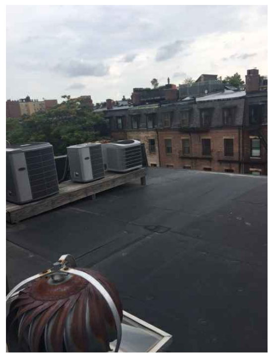
EXISTING ROOF TOP MECHANICAL UNITS
