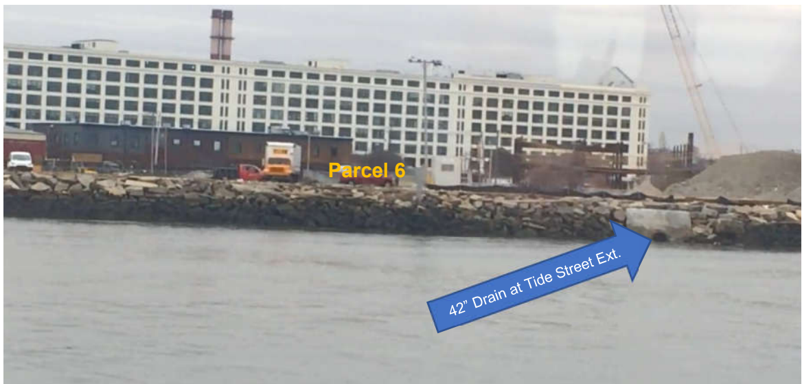
Site Photograph #1: Coastal bank from Boston Harbor looking south.
