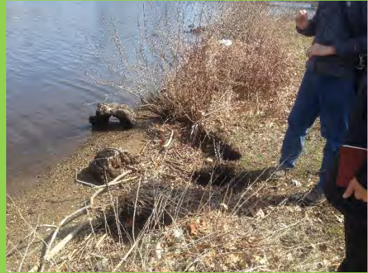
Figure 3--Eroded shoreline/proposed planting area
