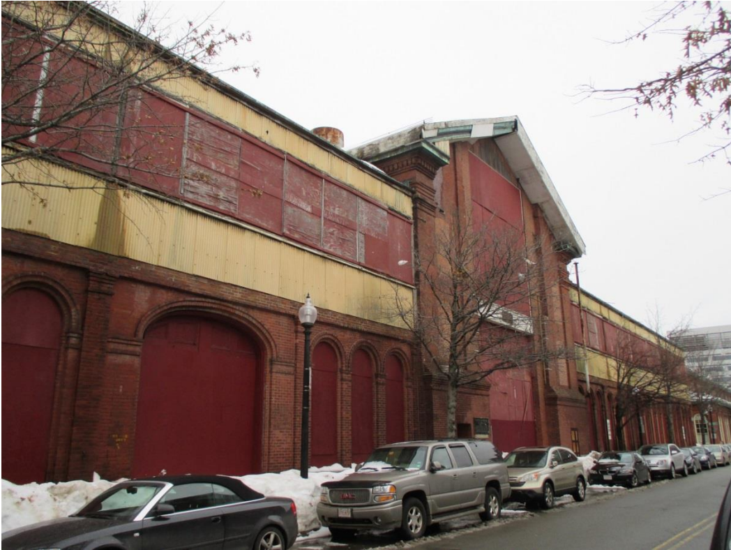
Photo 2: View facing north west from 1 st Avenue.
