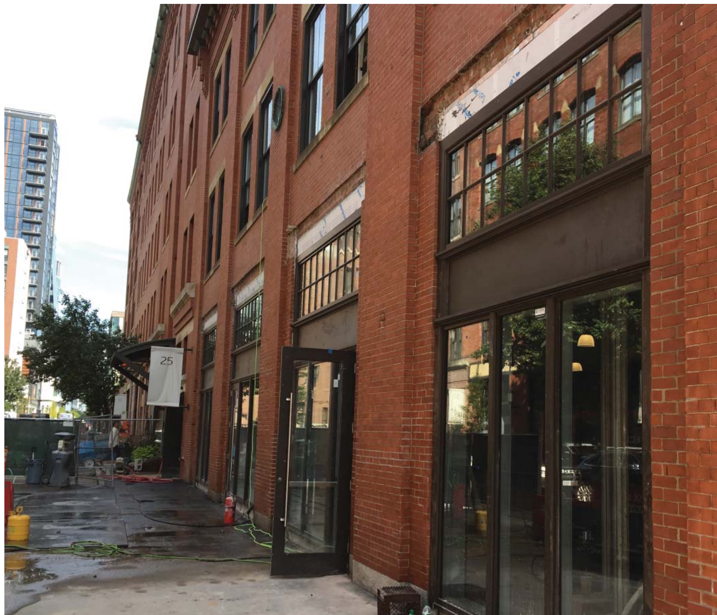
VIEW ALONG THOMSON PLACE
