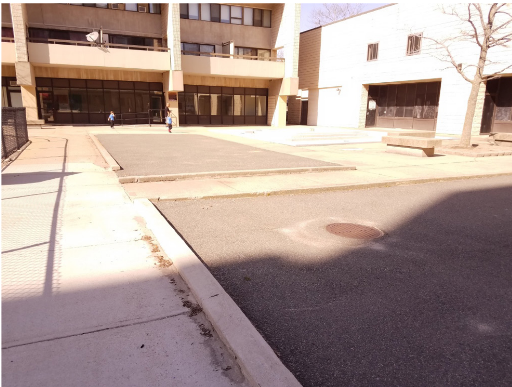
View of Existing Plaza and Concrete Area Looking North
