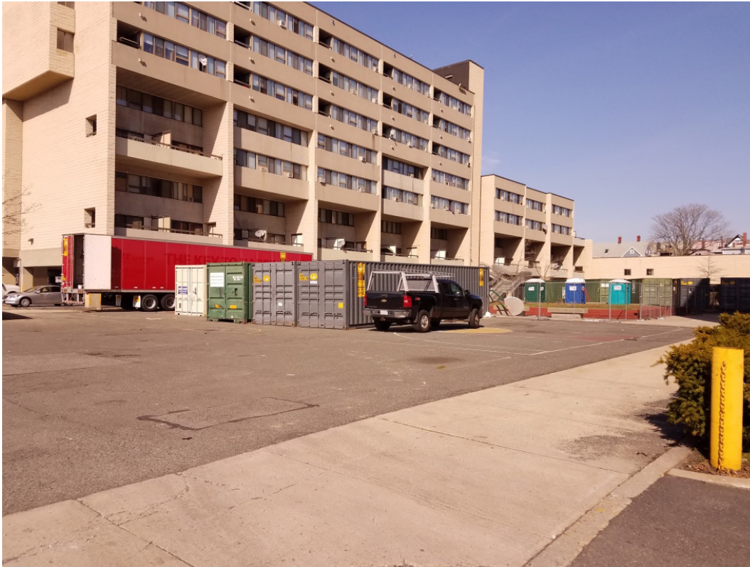
View of Existing Basketball Court and Concrete Area Looking North East
