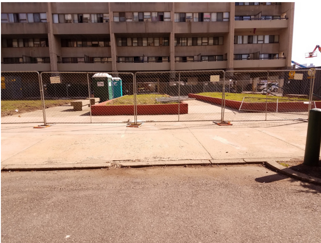
View of Existing Timber Planters Looking South
