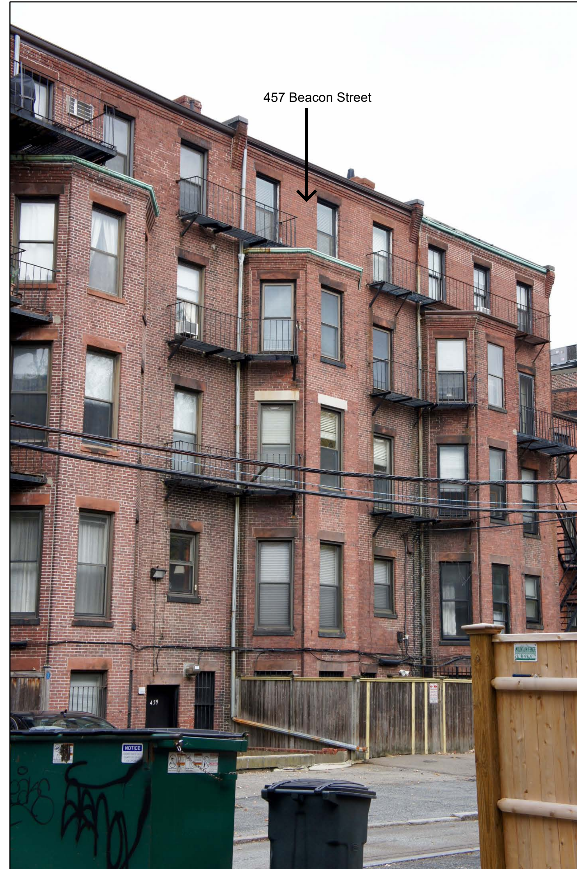
View Looking East of Rear of 457 Beacon Street from Public Alley 414
