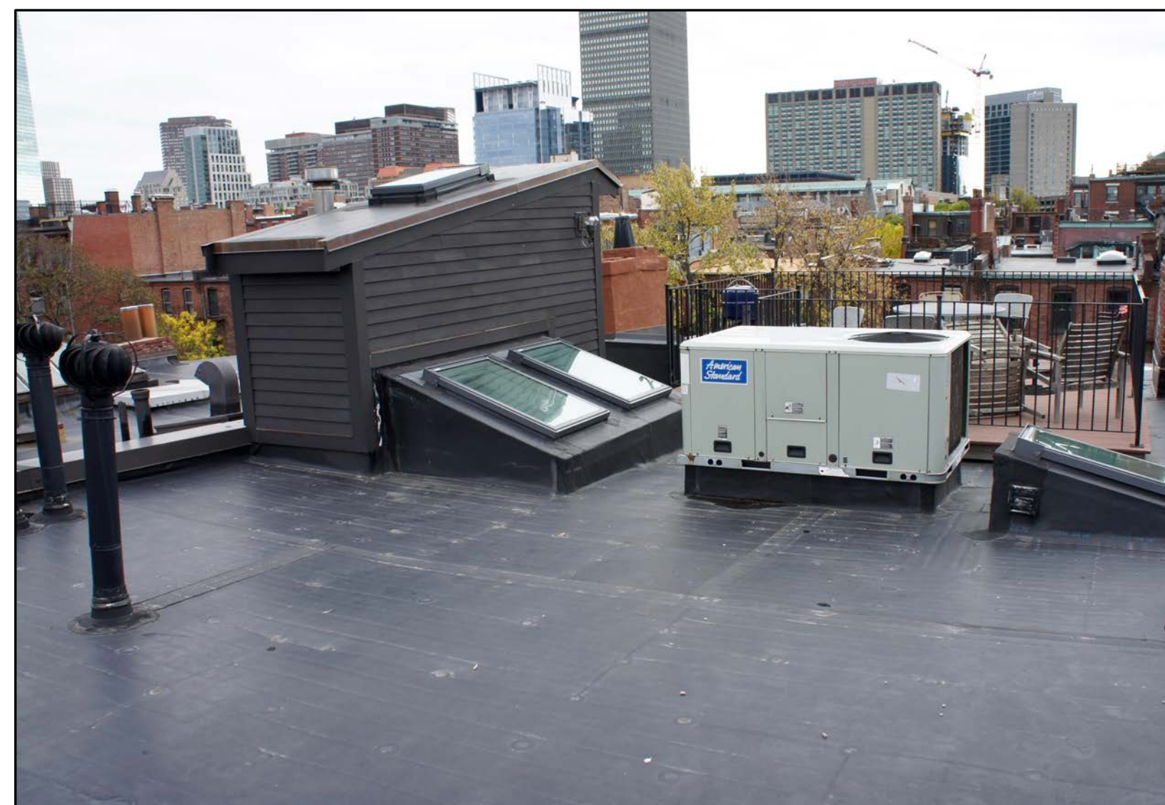
View of 457 Beacon Street Roof Looking Southeast
