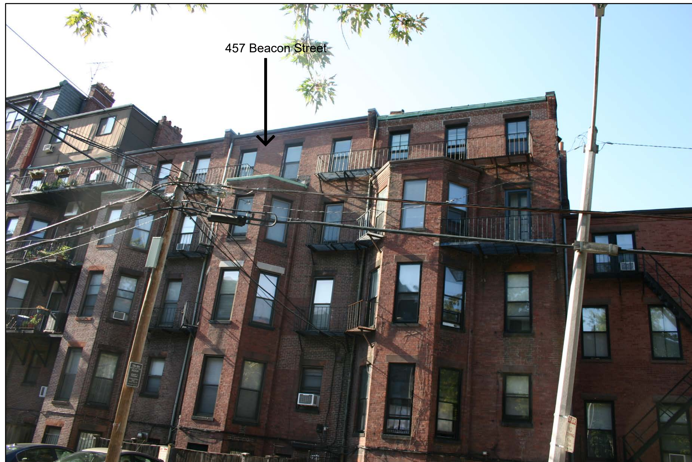
View Looking West of Rear of 457 Beacon Street from Public Alley 414
