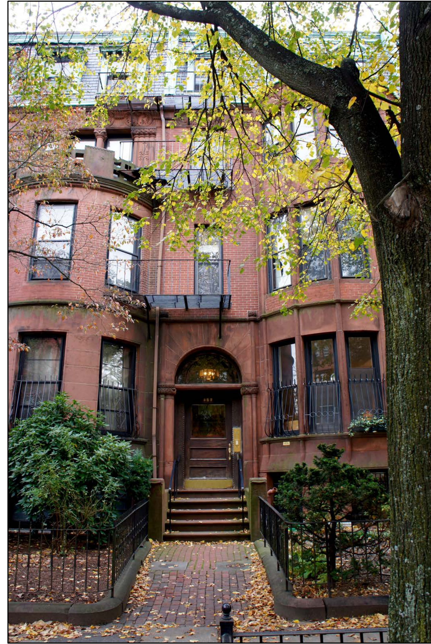
Beacon Street Facade Center View
