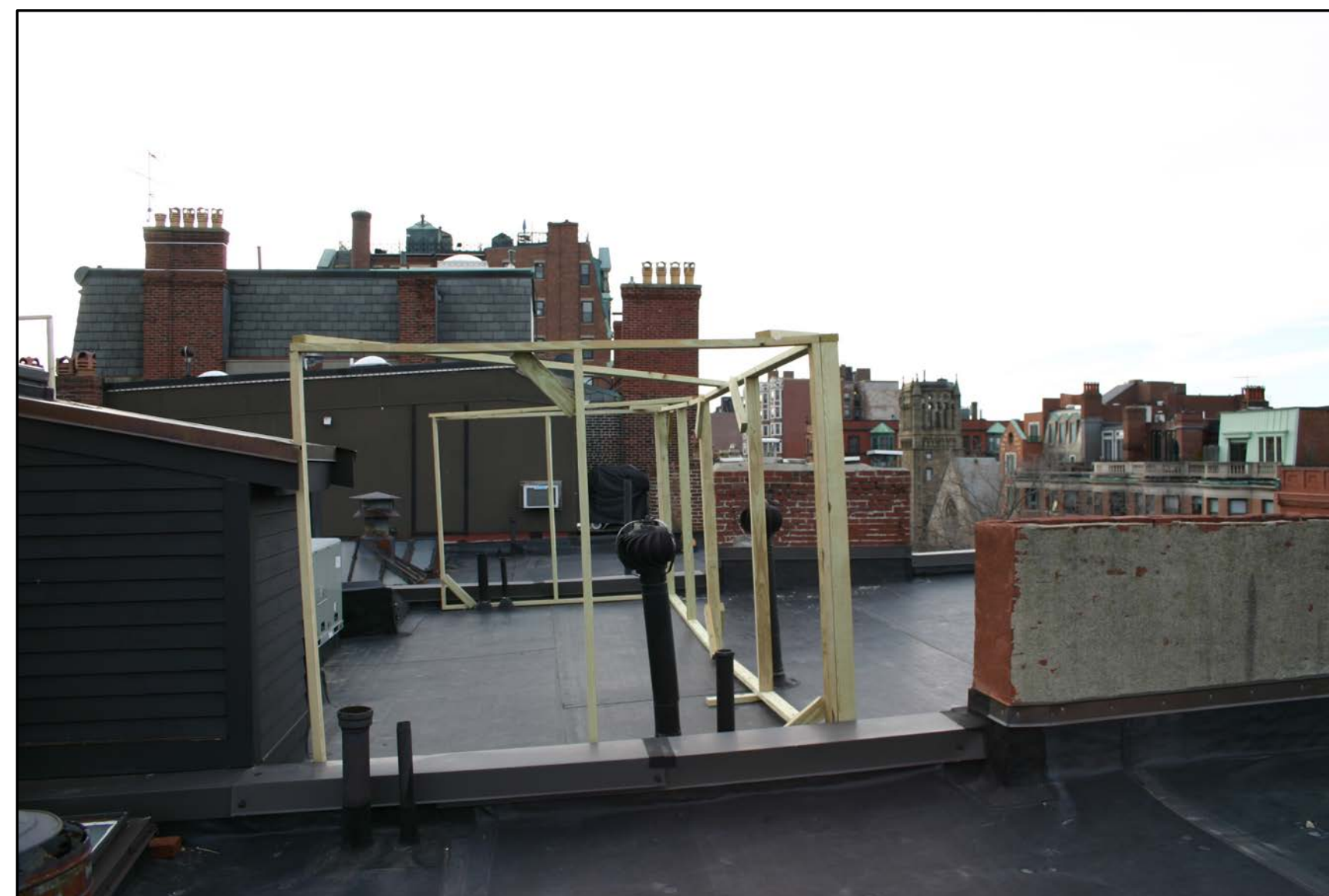
View of Front Mockup Looking West
