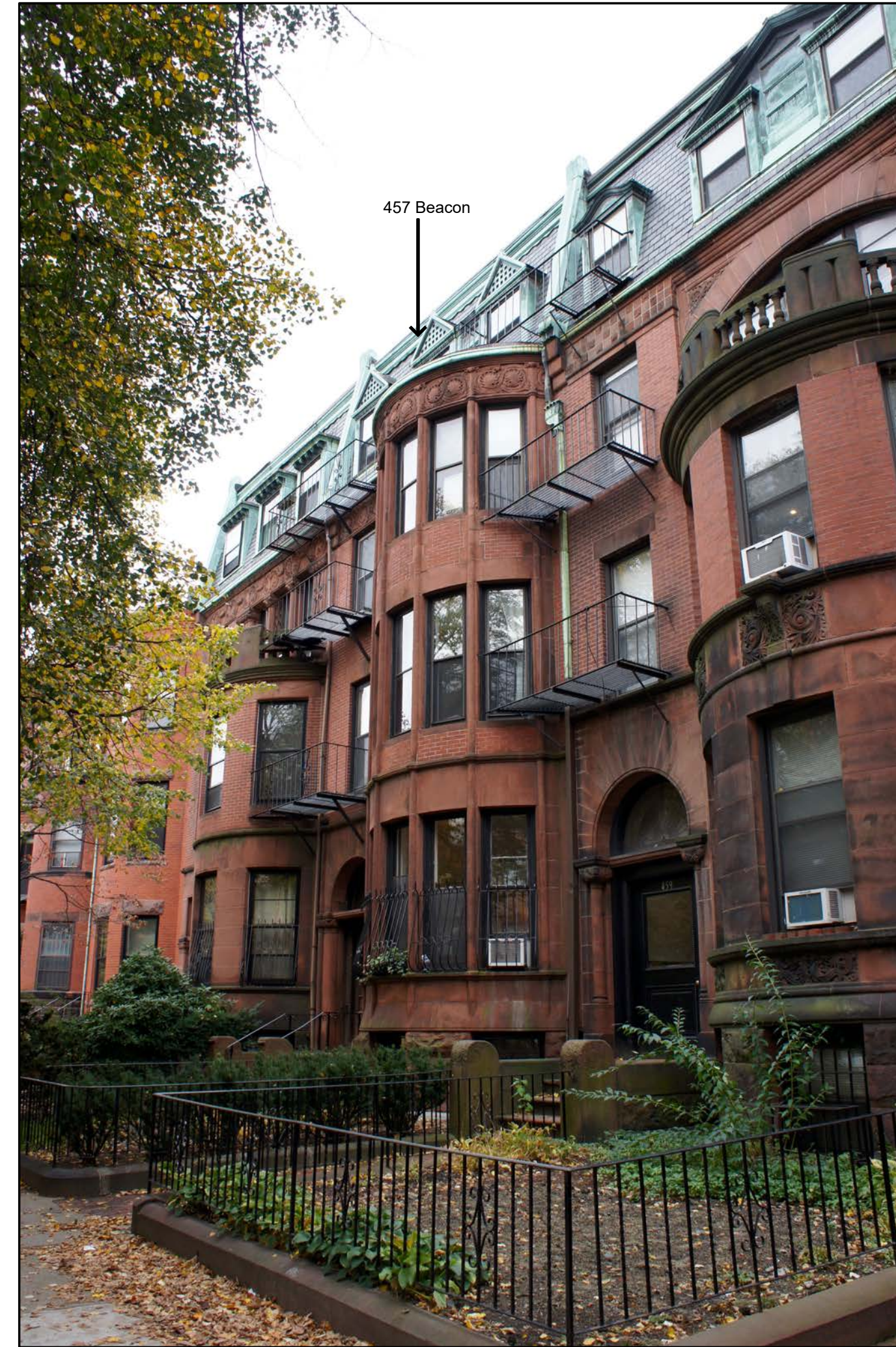
Beacon Street Facade Viewed from West
