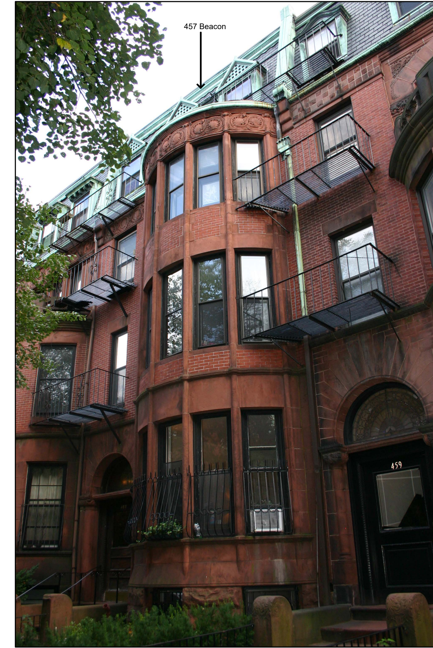
Beacon Street Facade Viewed from West
