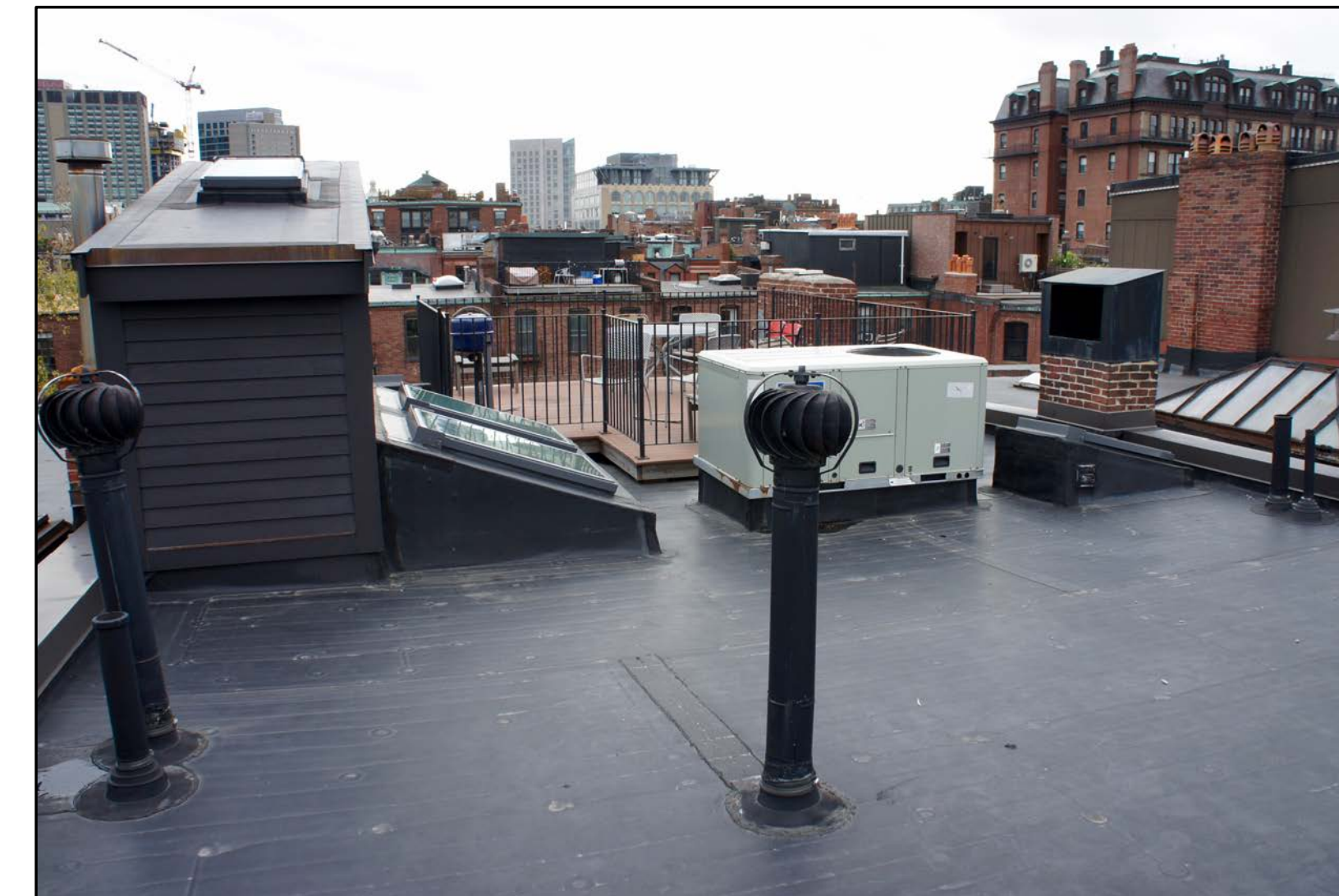
View of 457 Beacon Street Roof Looking Southwest
