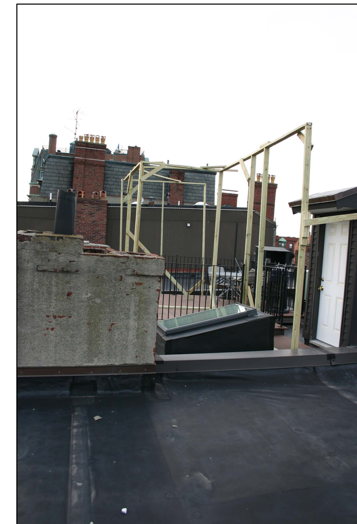
View of Rear Mockup Looking West
