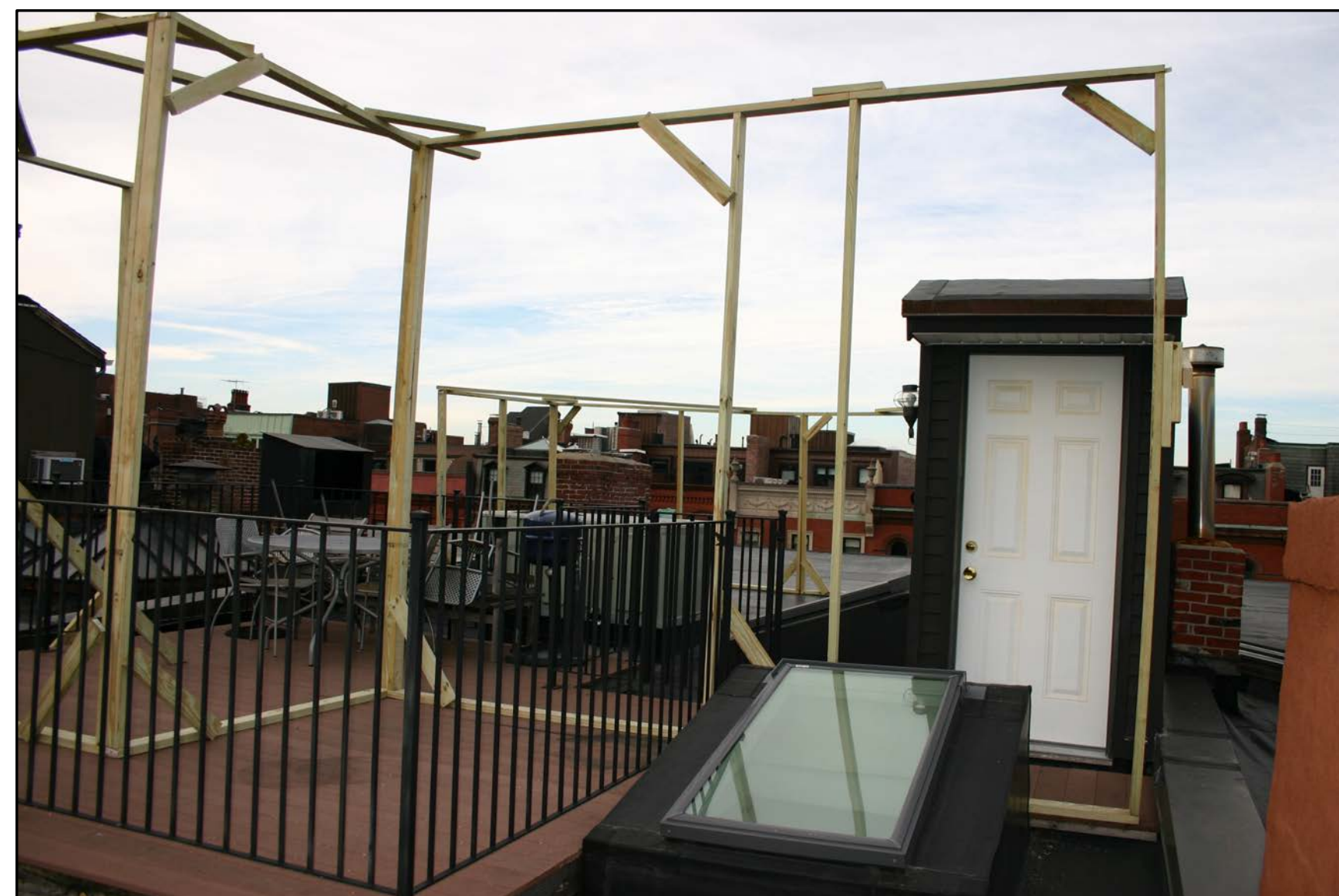
View of Rear Mockup Looking Northwest
