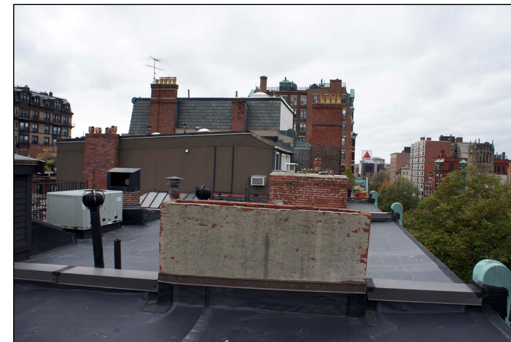
View of 457 Beacon Street Roof Looking West
