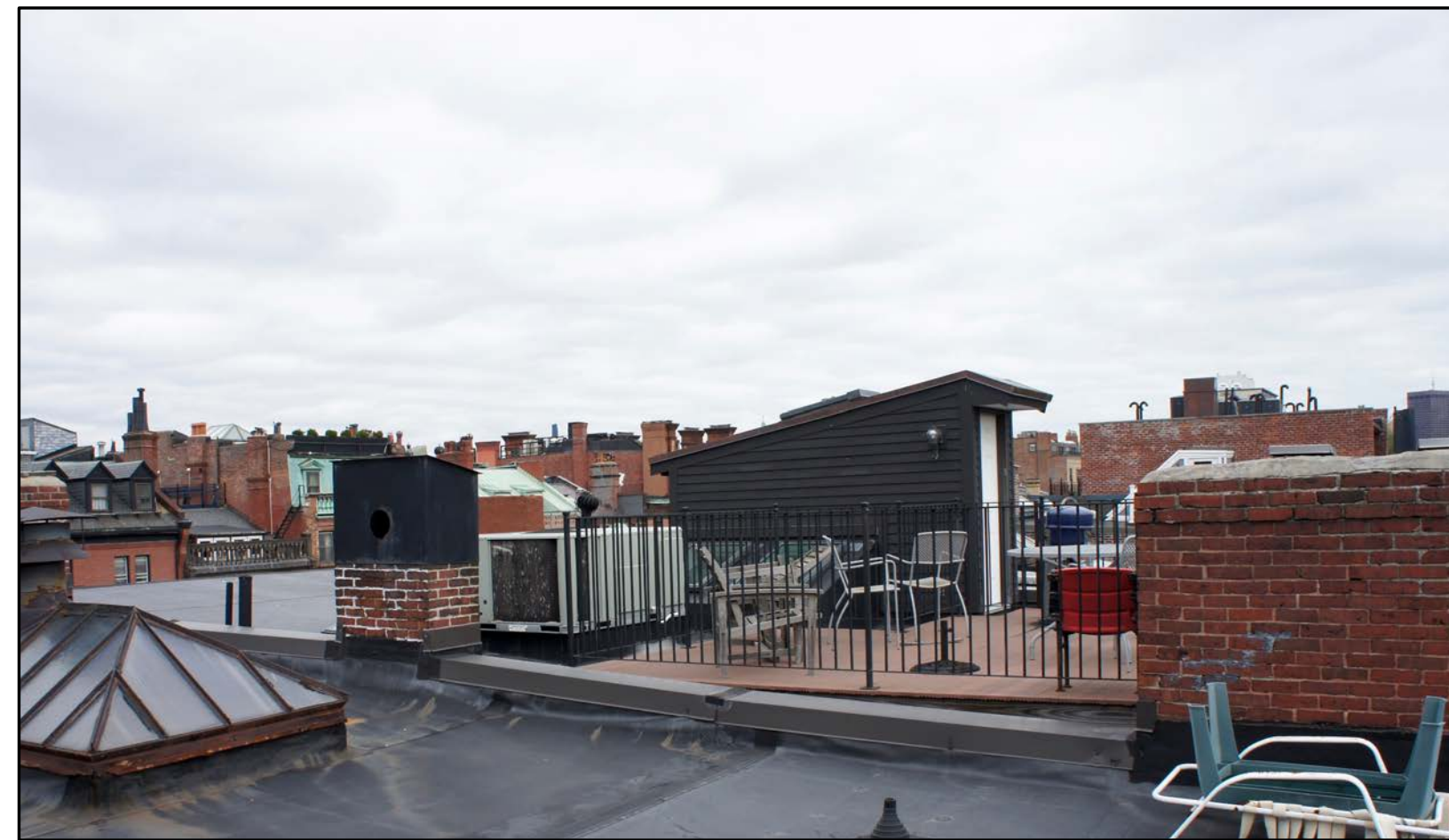
View of 457 Beacon Street Roof Looking Northeast
