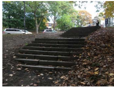
5 - Historic steps "A" and "B"
