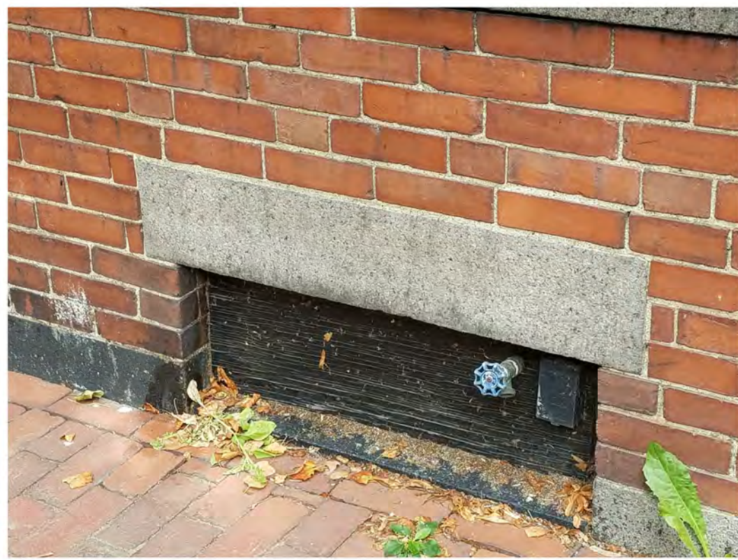
existing coal chute panel and spigot
