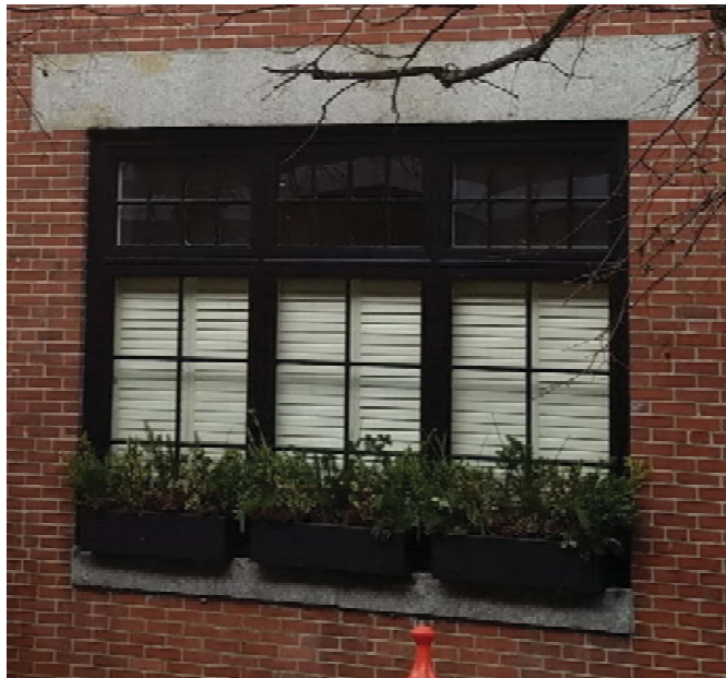
Detail: Neighboring existing windows at 85 Chestnut with six light windows below, 8 light transoms above
