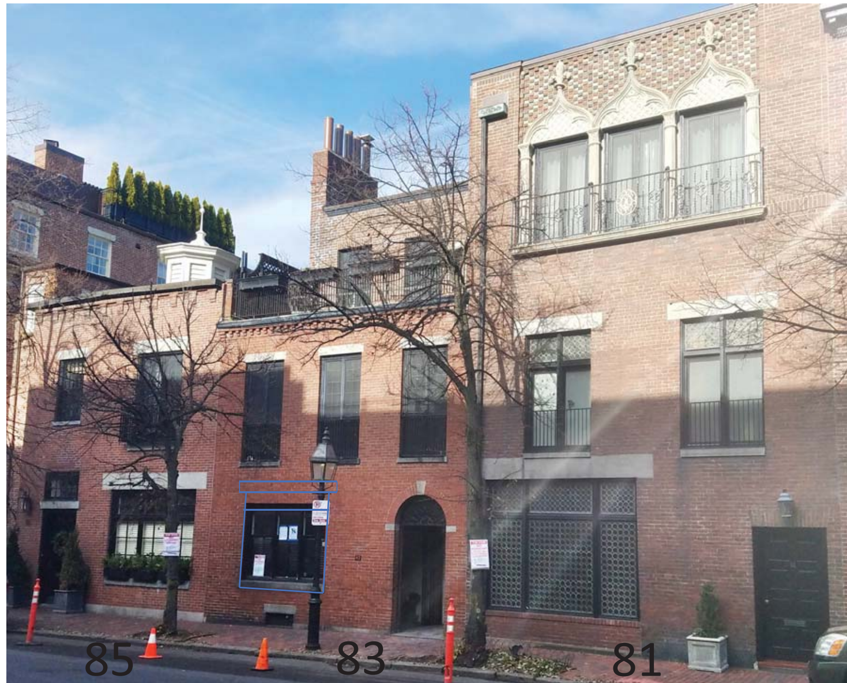
Overview: existing street level windows neighboring 83 Chestnut with proposed window enlargement to allow venting transom windows at top.
