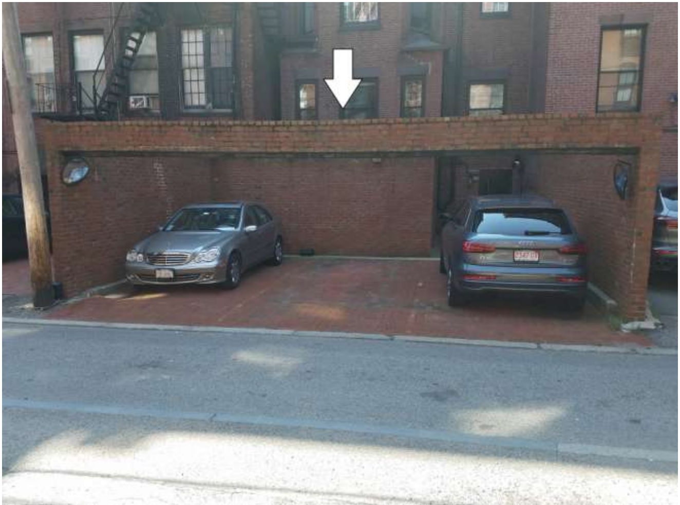
Photo below looks south across Public Alley 425 to the rear of 183 Comm Ave.
