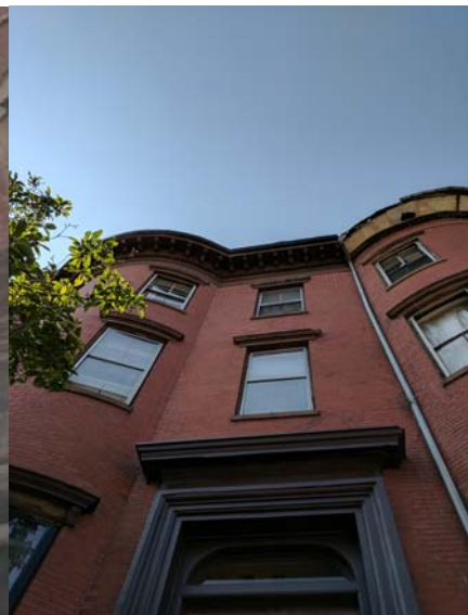
515 Mass Cornice to be Replicated
